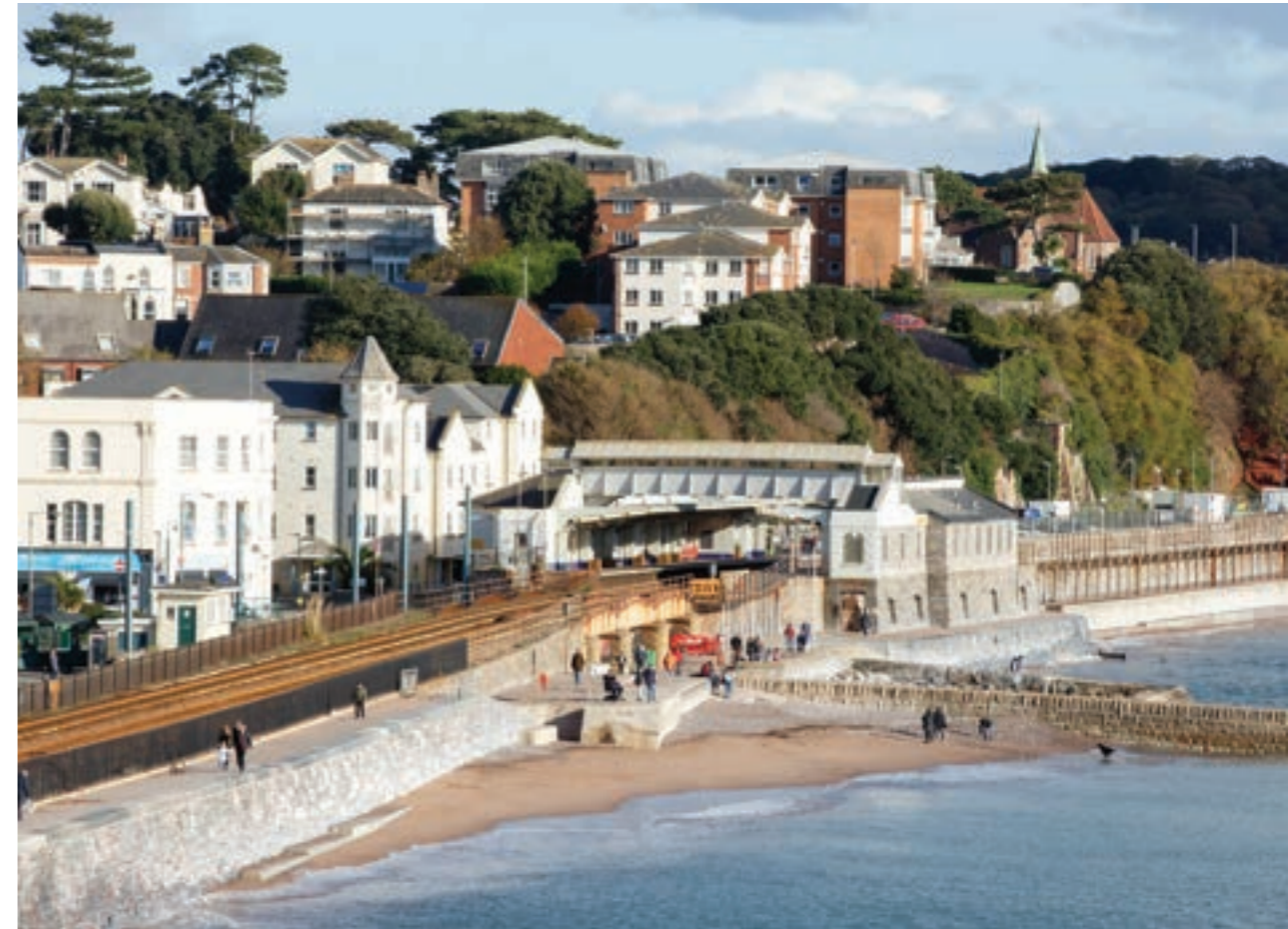
Dawlish has the first plastic footbridge to be listed Grade II for its architectural/historic significance. Designers specified the material, actually a high-tech Fibre Reinforced Polymer, to resist corrosion caused by the proximity of the English Channel at this Devon town.
