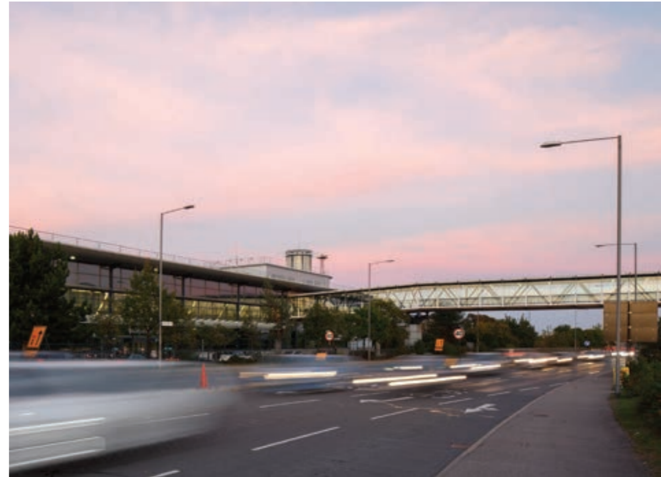
Ashford International, Kent, footbridge extends from the station across roads to a car park, all designed to be in harmony with the railway buildings.
