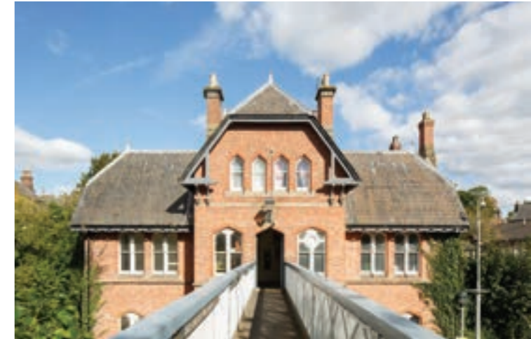
At Cressington, Liverpool, of 1864-73, listed Grade II for its special architectural/historic interest and restored by Network Rail's predecessor British Rail in the 1970s, the station has been arranged over three storeys, so that the footbridge emerges rather surprisingly from the first floor of the chalet-like building.
