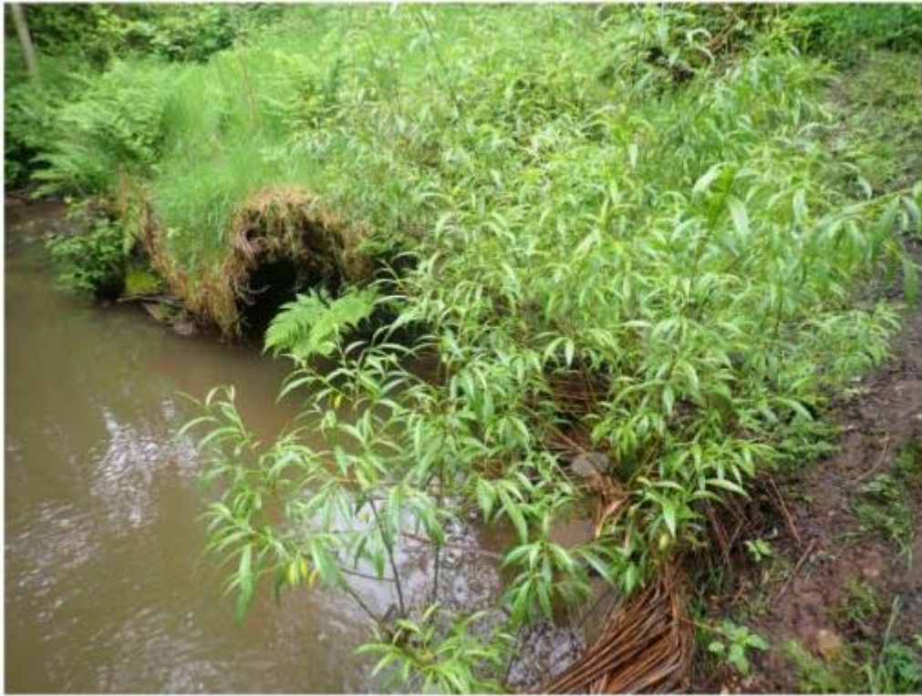
Figure 7: Living willow used to reduce scour
