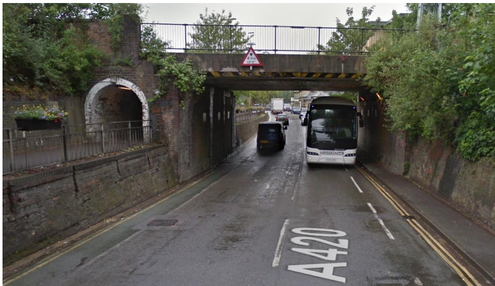
Figure 1: Original Botley Road bridge, looking west
