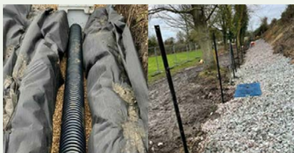
Catchpit and pipe runs and final re-instatement
