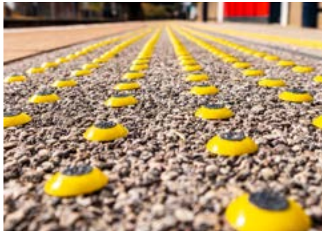
Image 4.3.2.1: AusTact composite tactile studs (Australia)
