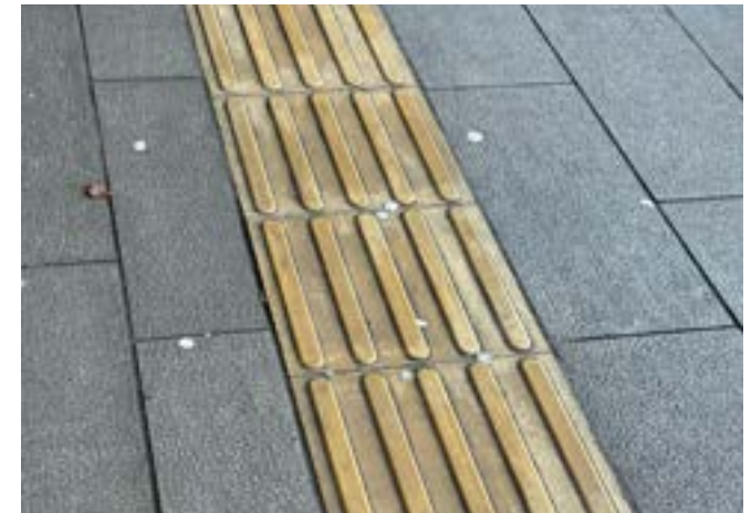
Image 2.3.1.2: Tactile guidance path at Coventry Station
