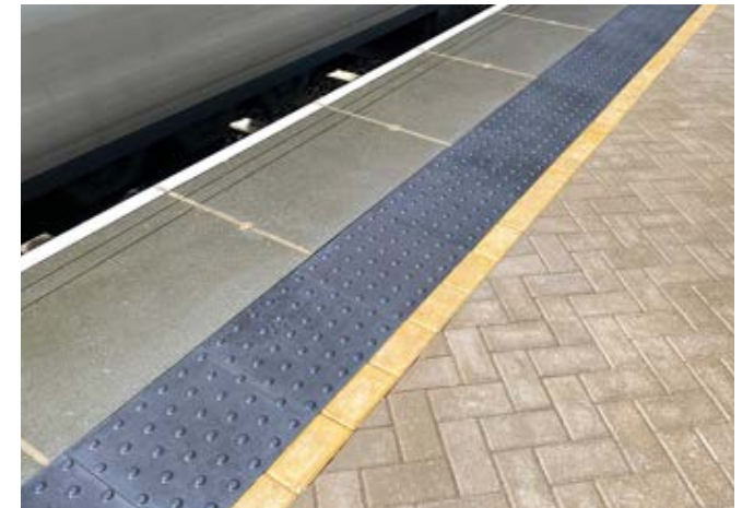
Image 2.2.2.2: Platform edge warning at Brent Cross West Station
