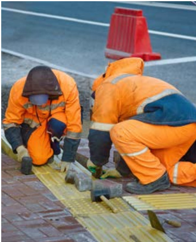
Image 1.3.1: Tactile paving installation
