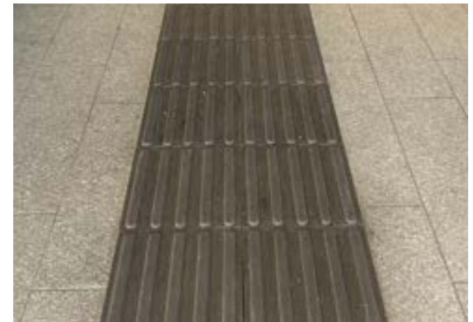
Image 2.3.1.3: Tactile guidance path at Barking Riverside Station
