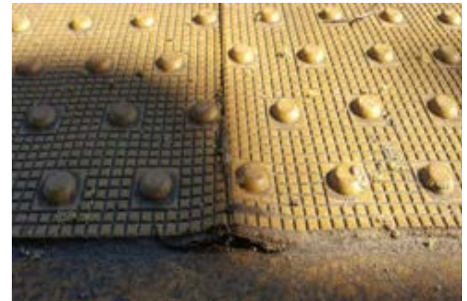
Image 4.3.4.1: Self-adhesive tiles should be avoided where a permanent installation is feasible
