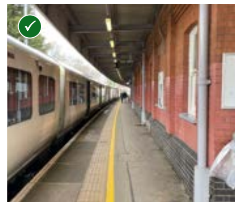
Image 2.5.5.2: If a tactile guidance path can not be installed on a platform, a continuous building line that is mainly unbroken could be used as a tapping feature
