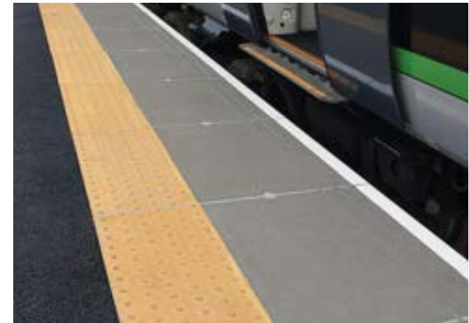
Image 4.7.1: Example of integrated platform edge coping and warning tactile, that are installed as single integrated product. (It is noted that this example is lacking a yellow line).
