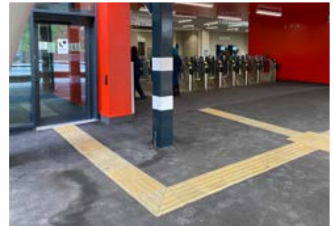
Image 2.4.3.2: Tactile guidance path leading to a waiting room
