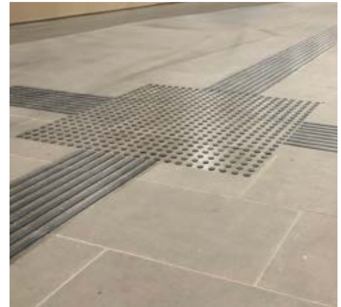
Image 4.3.1.7: Surface-mounted adhesive studs
