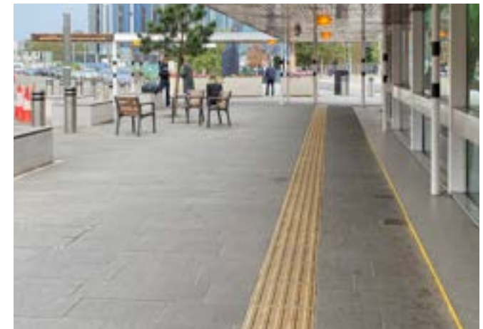
Image 2.4.4.2: External tactile guidance path at Coventry Station
