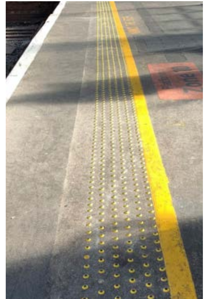
Image 4.3.2.3: AusTact composite studs installed at York Station
