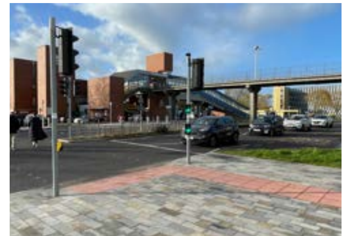
Image 2.2.4.3: Controlled pedestrian crossing, Stevenage
