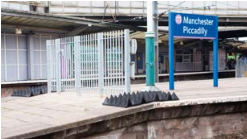
Image 3.1.3.1: Platform fitted with a security gate and rubber anti-trespass panels
