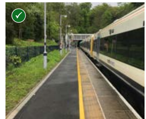
Image 2.5.5.3: If a tactile guidance path can not be installed on a platform, a kerb or fence that runs parallel to the platform could be used as a tapping feature
