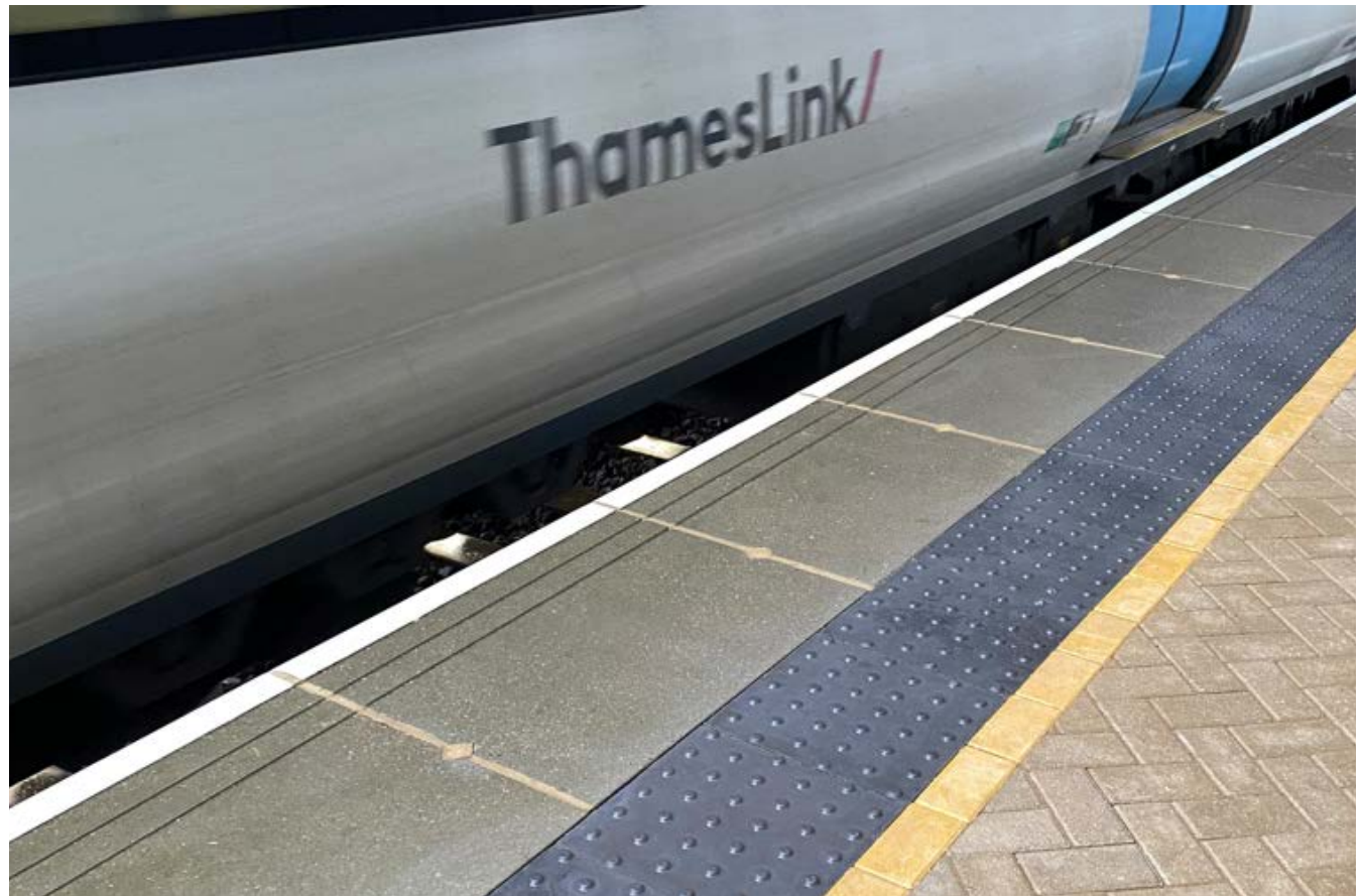
Image 4.3.1: Concrete platform edge warning tactile
