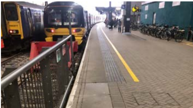
Image 3.1.4.1: Platform fitted with a protective barrier leading onto a platform
