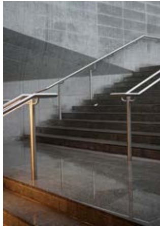
Image 9.3 Granite walls, floors and steps
