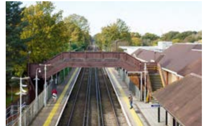
Image 7.2 Timber bridge at Martins Heron station
