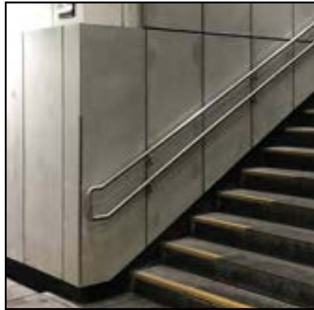
Image 9.4 Concrete element wall cladding elements
