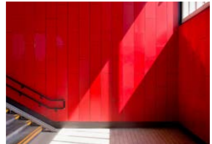
Image 9.10 – Metal Cladding Panels Strong use of colour, and vertical staggered arrangement
