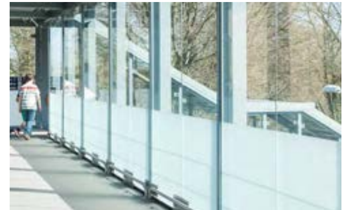
Image 7.9 Transparent glass with lower section obscured..
