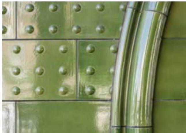
Image 9.9 – Ceramics, Faience tiles Bold faience tiles used with relief designs in a contemporary interpretation of a traditional material
