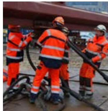
Image 5.19 Preparing the hoist
