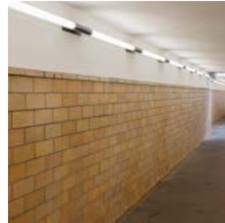
Image 9.5 Ceramic tile wall cladding
