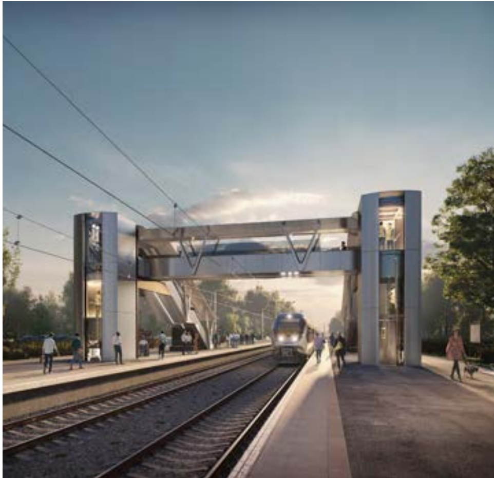
Image 4.35 AVA in a covered standard version seen from the back expressing the use of stainless steel.
