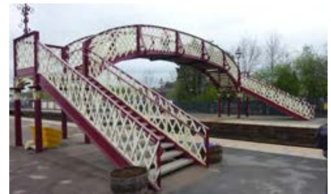
Image 6.9 Listed bridge in Appleby station that was salvaged from another station.
