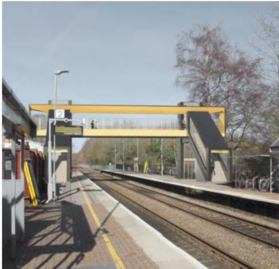
Image 4.20 Frame in a covered standard version seen from the front with its characteristic yellow frame.
