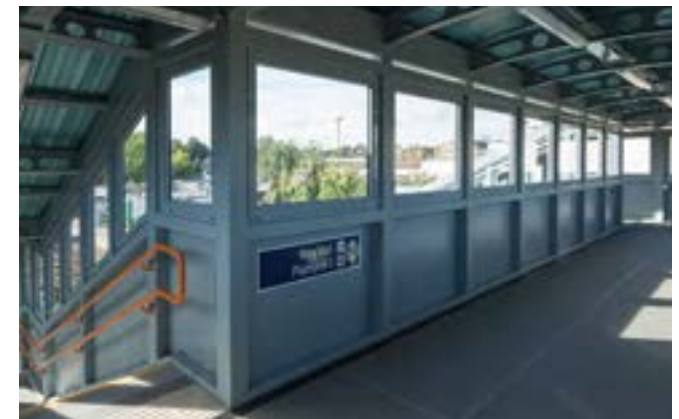
Image 7.24 Internal view of Alton station footbridge.
