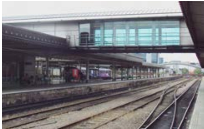
Image 6.14 Sheffield station — external walkway for maintenance
