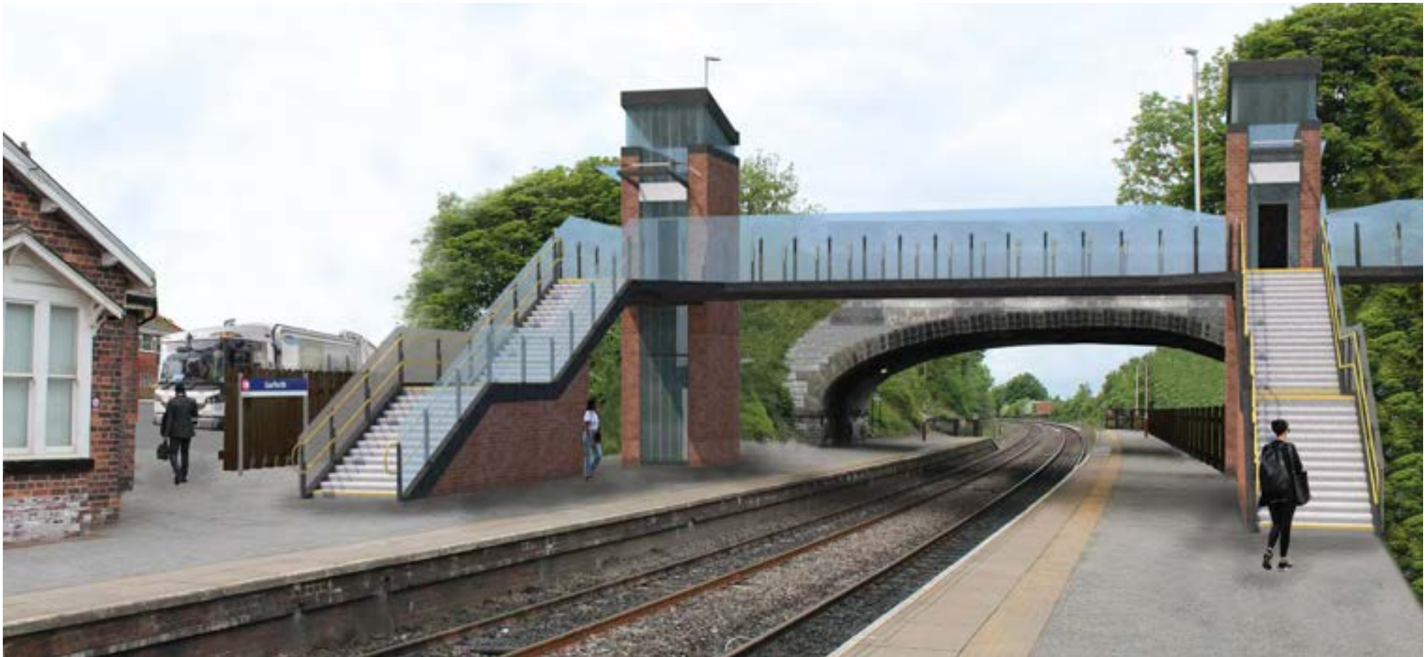
Image 4.10 Visualisation of the Beacon footbridge without roof cover, fully glazed for maximum visibility and with solid brick basis in technical rooms and lifts.
