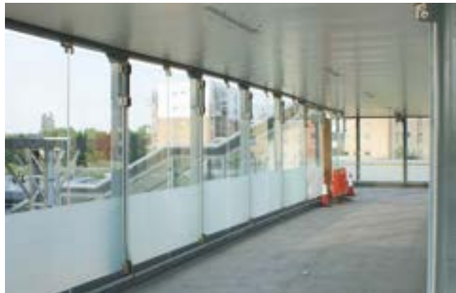
Image 6.15 Cambridge station — inwardly openable glass panels
