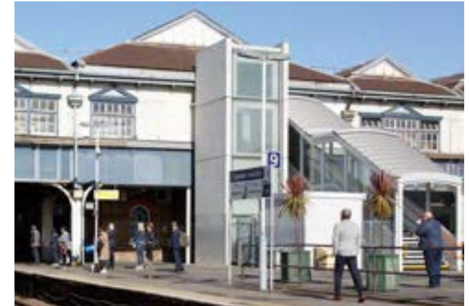
Image 6.7 Modern materials and detailing. At Clapham Junction station lift shafts and new staircases have been fitted to the existing footbridge.
