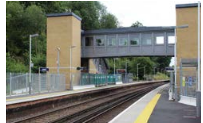
Image 6.16 Godalming station — glazing at high level only
