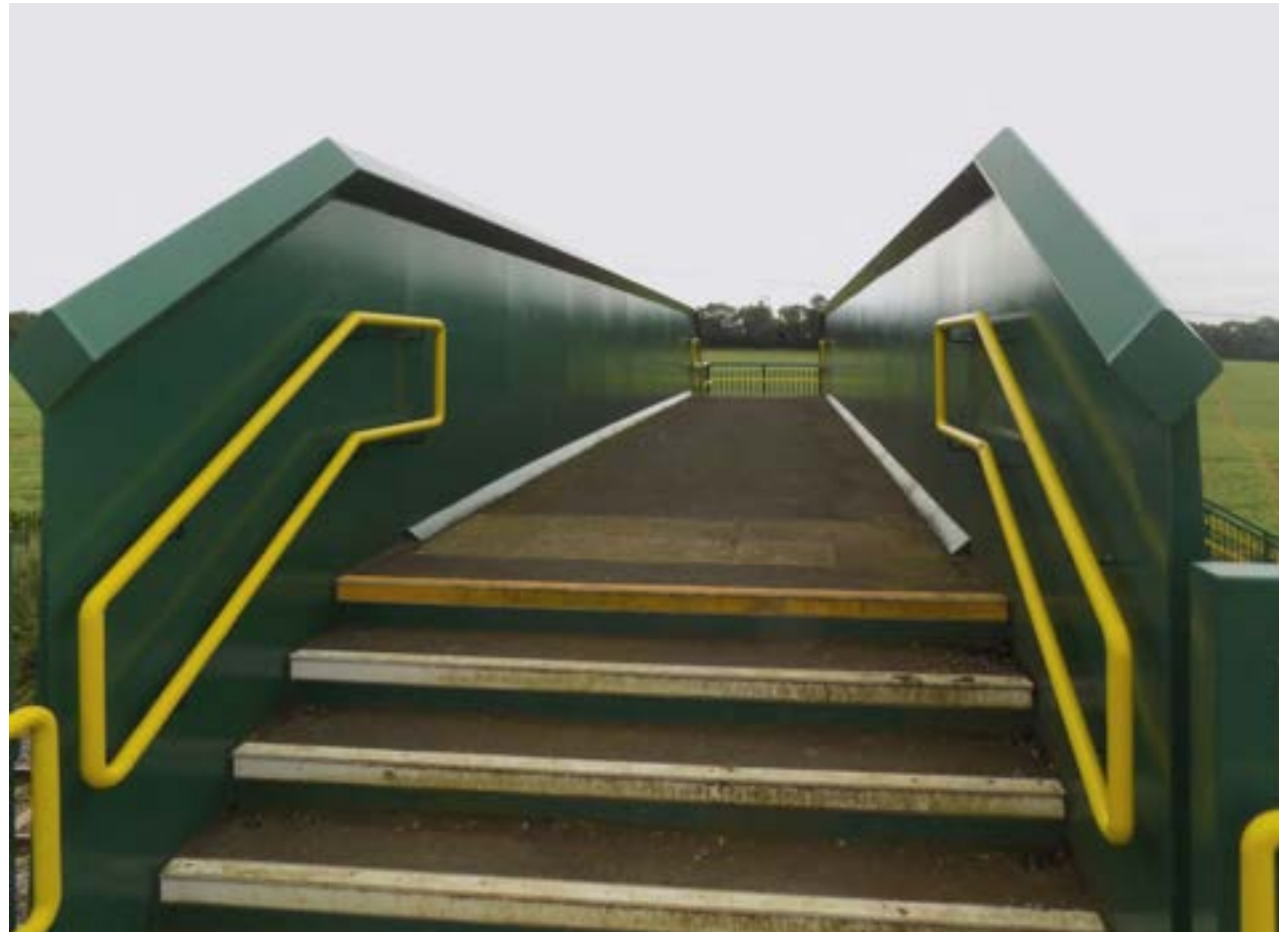
Image 5.5 Enclosed bridge sides at Wymington footbridge.
