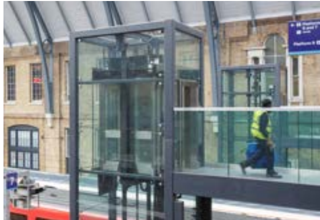
Image 6.6 Modern approach to differentiate new additions. At King's Cross station the lift shafts have a modern simple aesthetic, with colour tying the lifts to existing structure.
