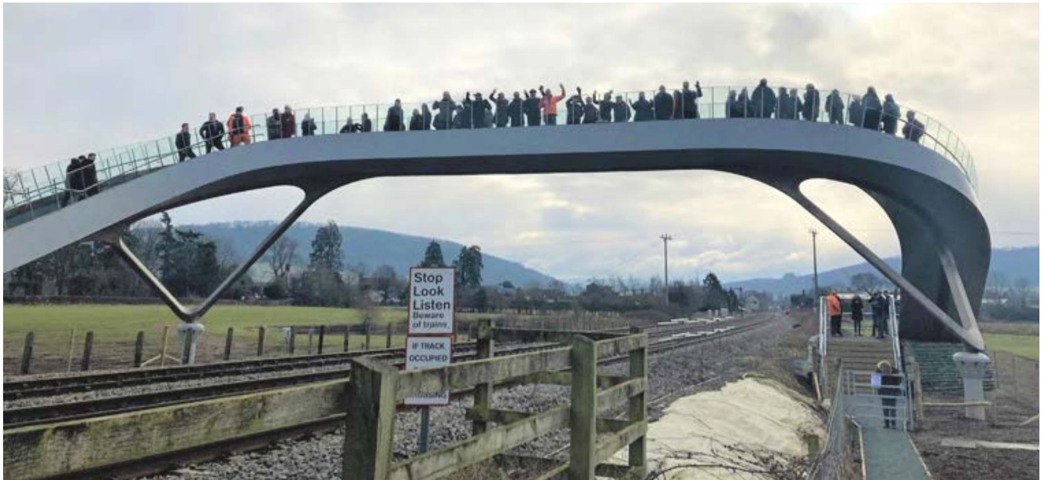
Image 5.10 Flow bridge where pedestrians are easily visible due to the use of glass on the sides of the bridge.
