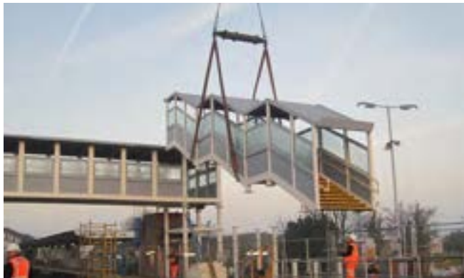
Image 6.21 Staircase being craned into place at Sittingbourne station.
