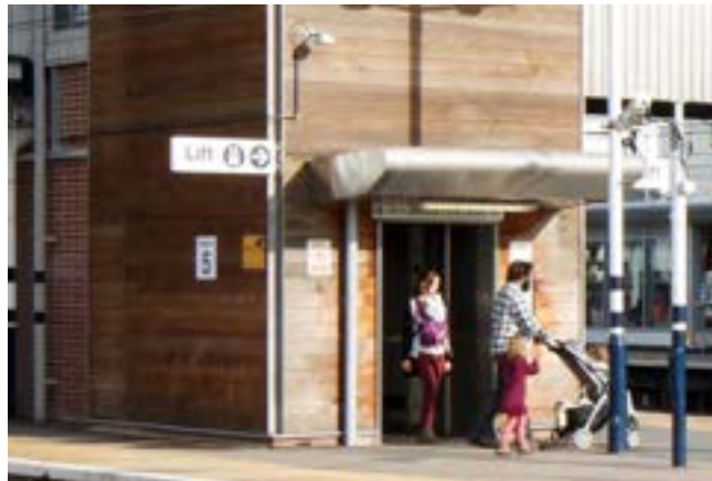
Image 7.4 Timber clad lifts in Peterborough Station.
