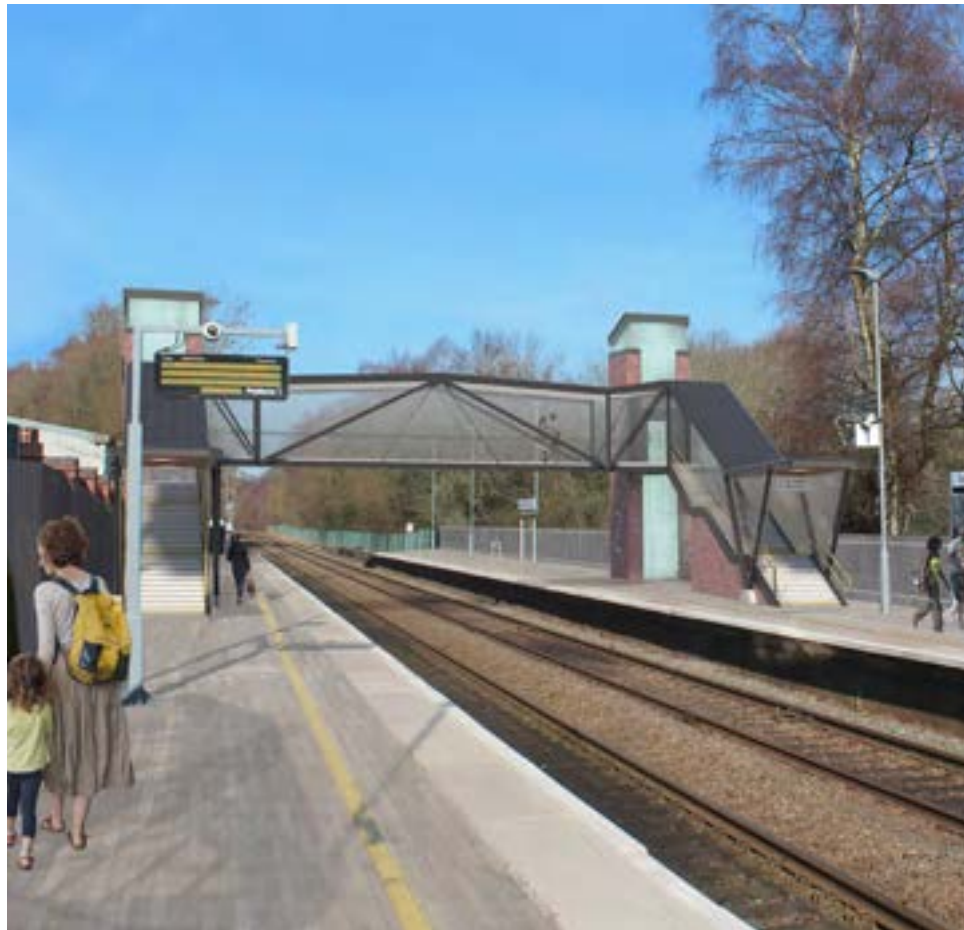
Image 4.3 Beacon in a covered standard version stands out with its fully glazed sides on bridge and stairs.
