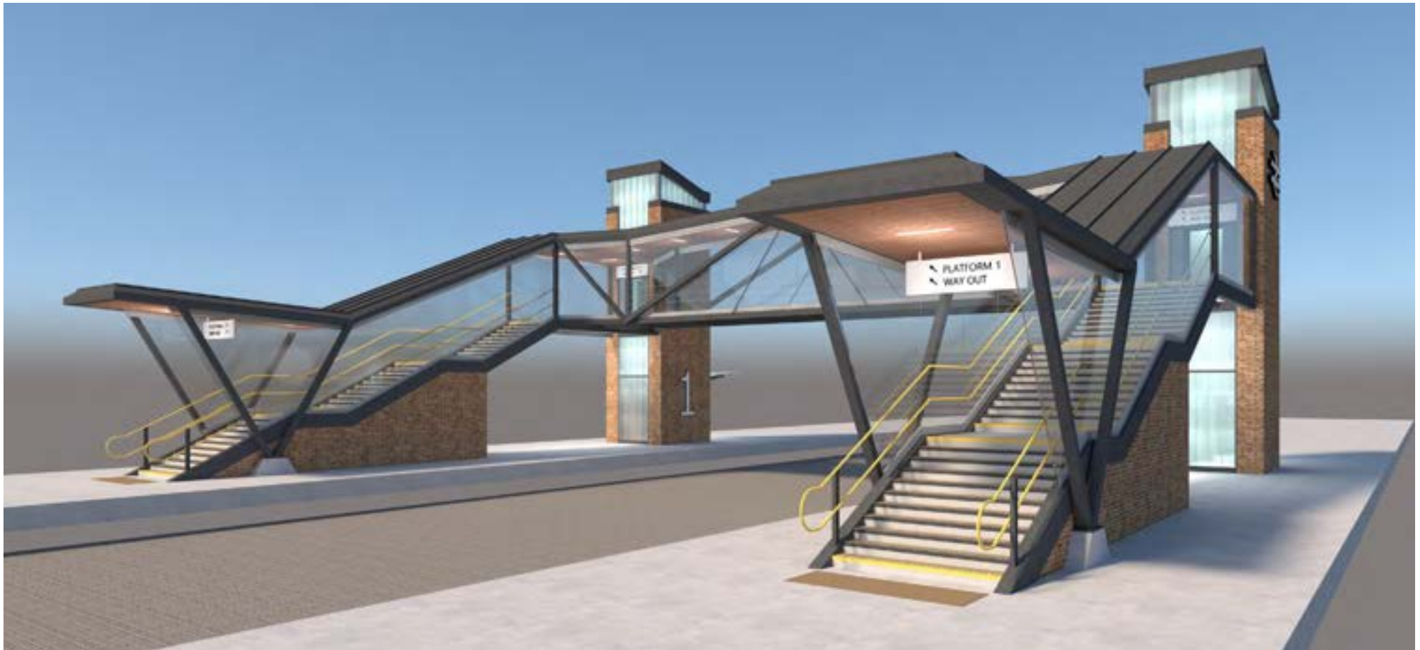
Image 4.5 Visualisation of the Beacon footbridge. Fully glazed for maximum visibility and with solid brick basis in technical rooms and lifts.
