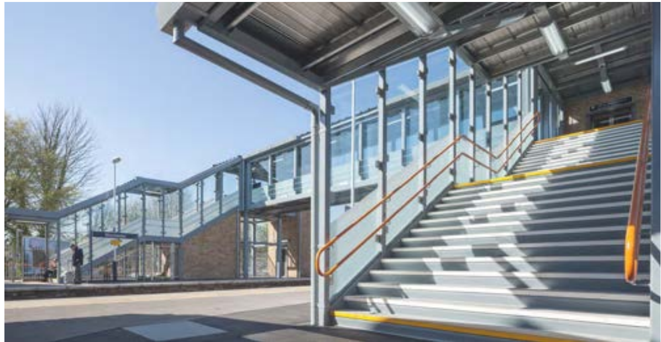
Image 7.13 Staircase at Winchester station.
