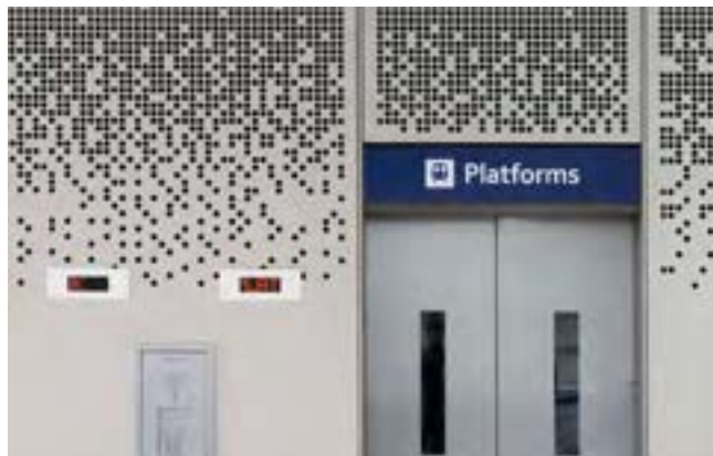
Image 7.6 Metal Cladding panels in Paddington Station.
