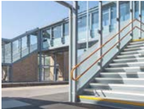
Image 1.8 A fully glazed and covered footbridge
