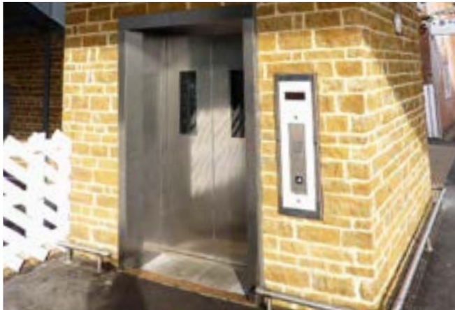
Image 6.5 Using Traditional Materials. Stone facing detailing to new lifts at Wellingborough station.
