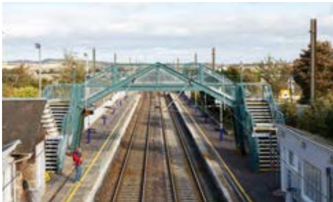
Image 6.12 Example of footbridge over OHLE at Drem Station
