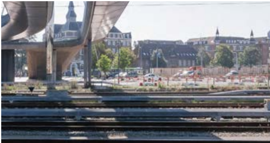
Image 5.15 A footbridge crossing the tracks
