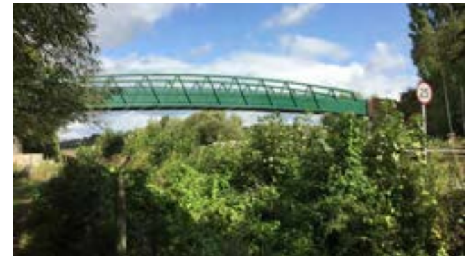
Image 6.8 Aristotle Lane, Oxford. The form and colour of this public crossing footbridge blends well into the landscape and is barely noticeable from a distance.
