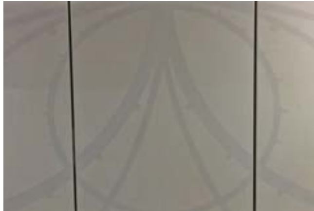
Image 9.7 – Vitreous Enamel Large format openable panels with a striking graphic motif screen printed onto the panel before baking.
