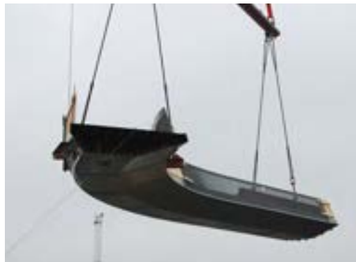
Image 5.18 Hoisting a footbridge into position
