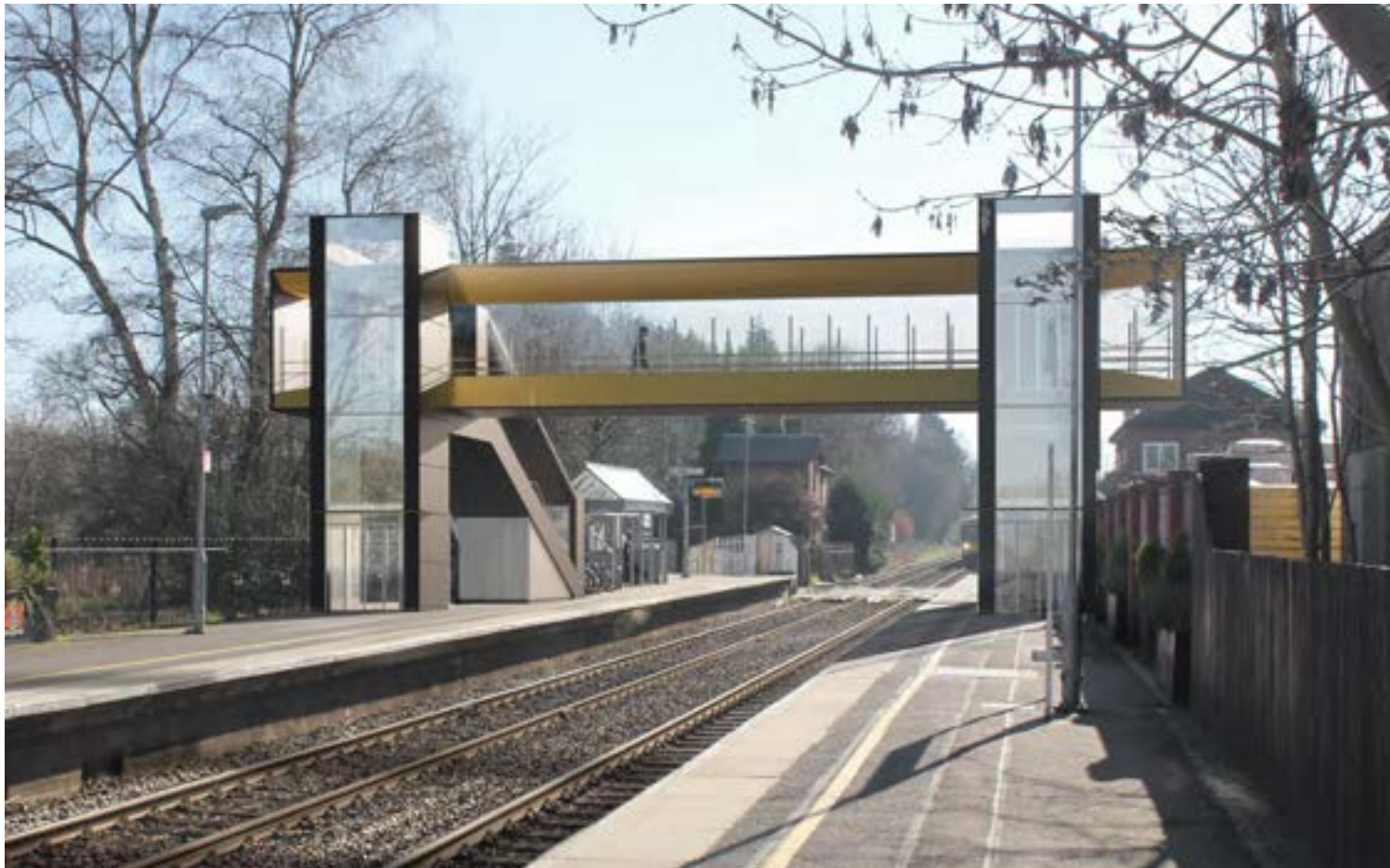
Image 4.22 Frame in a covered standard version seen from the back with the cantilevered wings on either side of the transparent lift towers.
