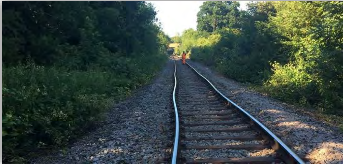
Figure 4.3-2: Track buckle on Western route in summer 2018.
