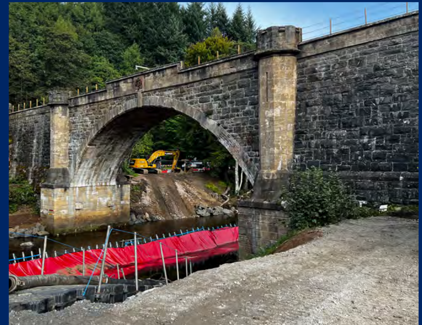
Inver viaduct, Dunkeld (2023)
