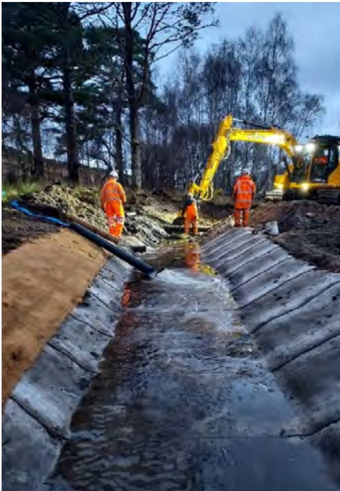
Drainage ditch / channel renewal
