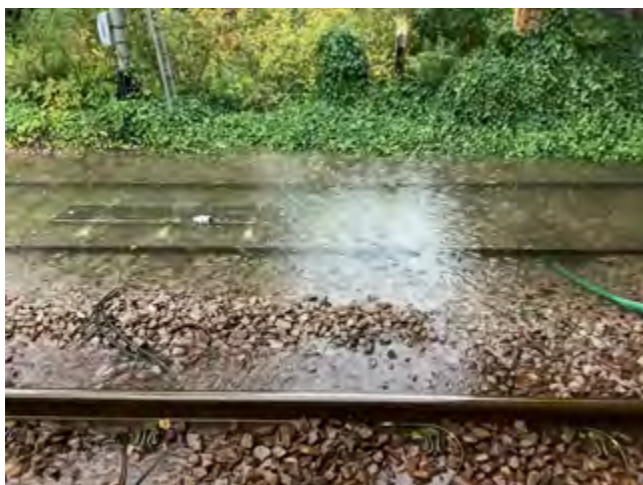
Track flooding
