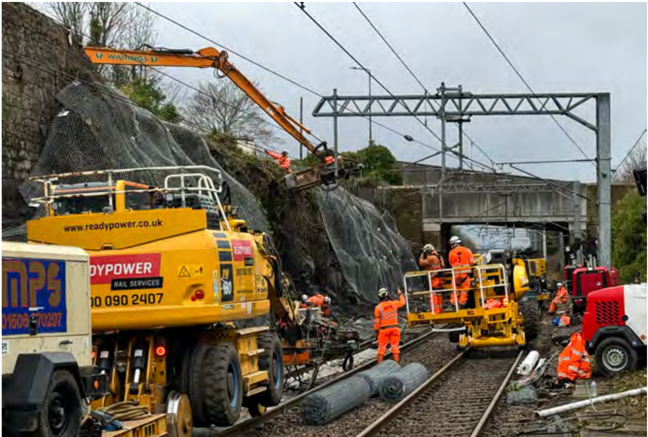
Installation of rockfall prevention measures at Ratho (2024)
