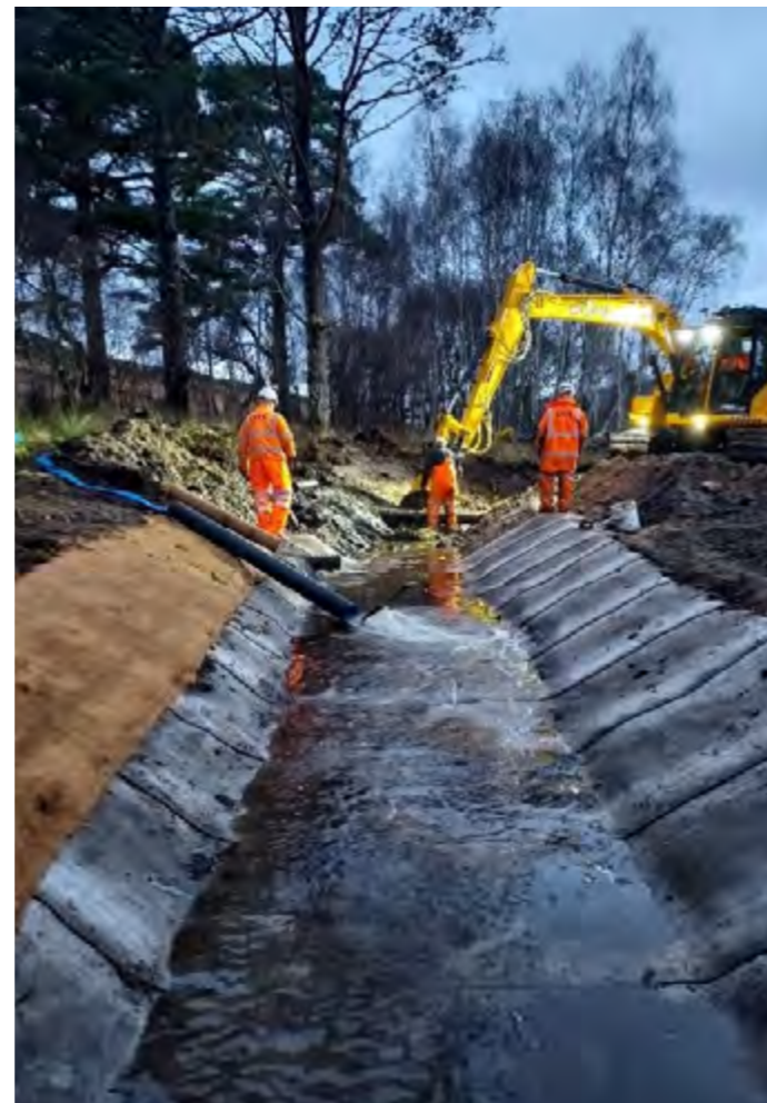
Drainage ditch / channel renewal
