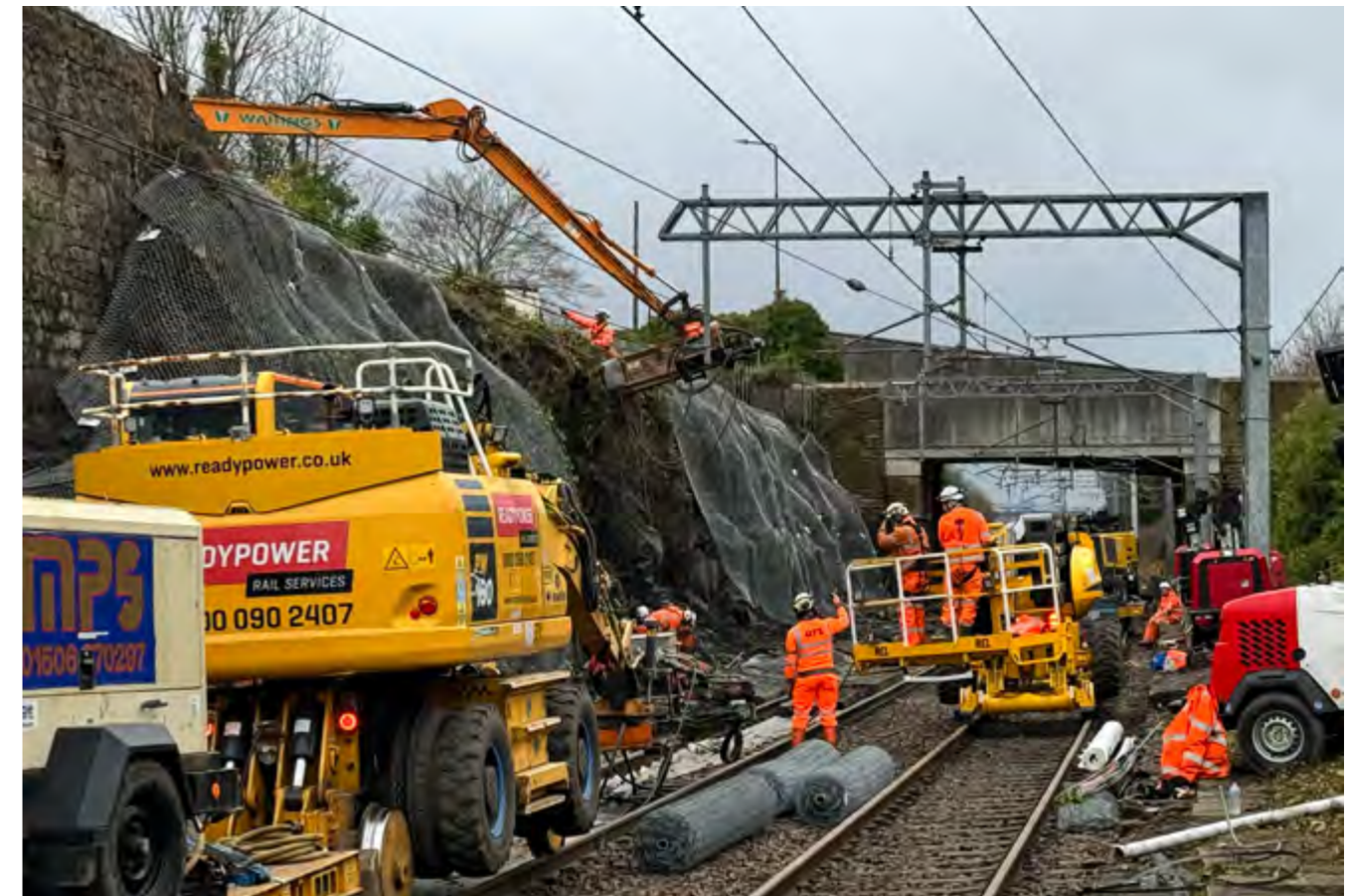
Installation of rockfall prevention measures at Ratho (2024)
