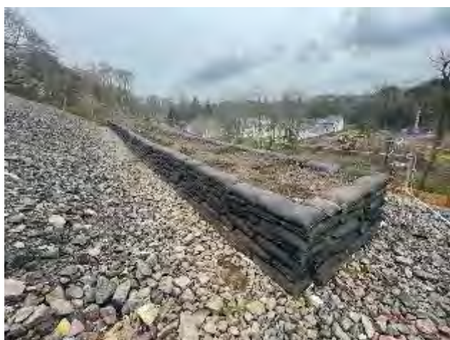
Figure 172: Raised beds installed as part of the Fairlie landslip remediation
