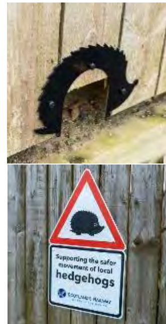
Figure 150: Hedgehog hole installed in the fence along with signage
