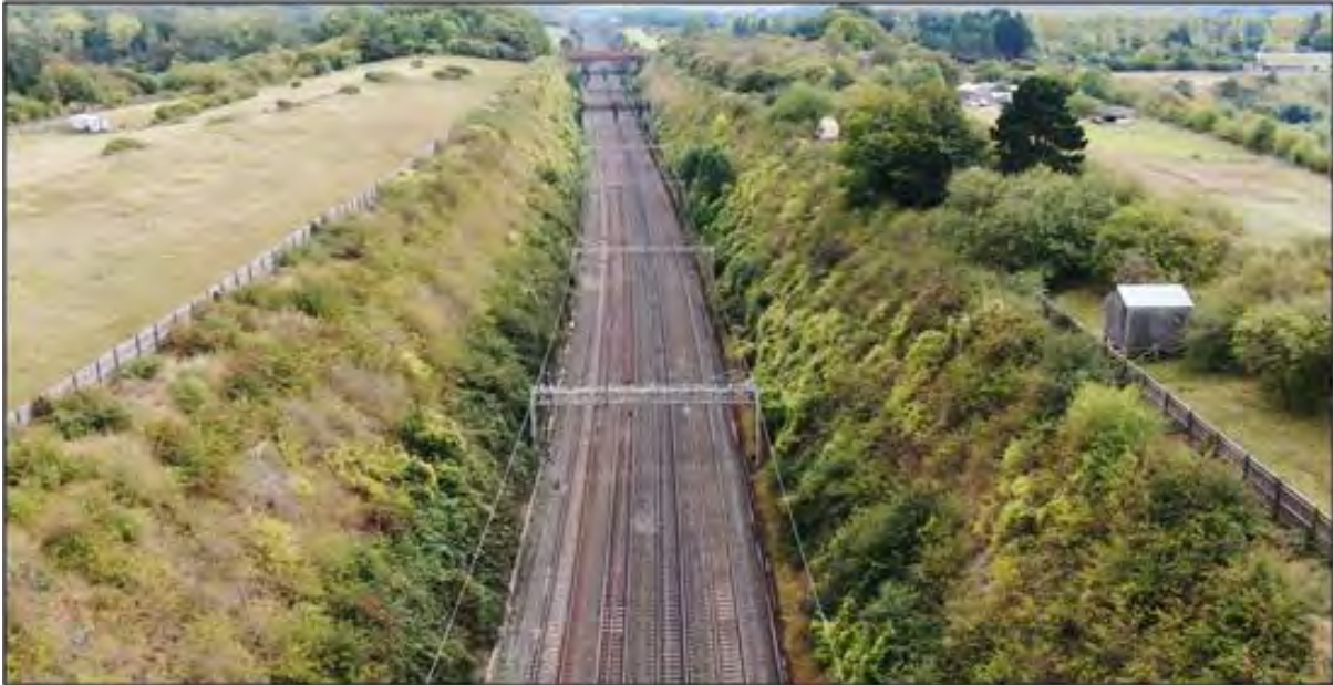
Figure 6: Still from drone footage (facing south at approx. 33.0671 M.Yds) prior to vegetation management
