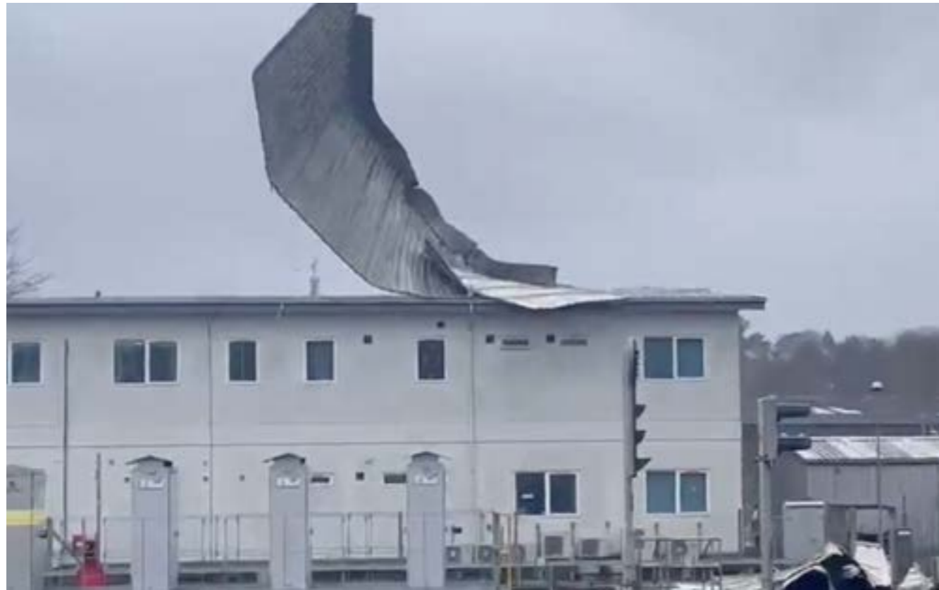
Figure 24) A network rail delivery unit roof blows off during Storm Eunice – resulting in Chiltern Railway services being suspended. Source: https://twitter.com/networkrail/status/1494697757684215812?lang=en Credit: Chilterns Railway.
