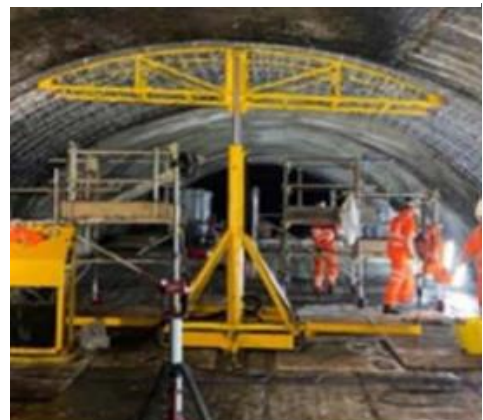
Figure 3. Tunnel repair work
