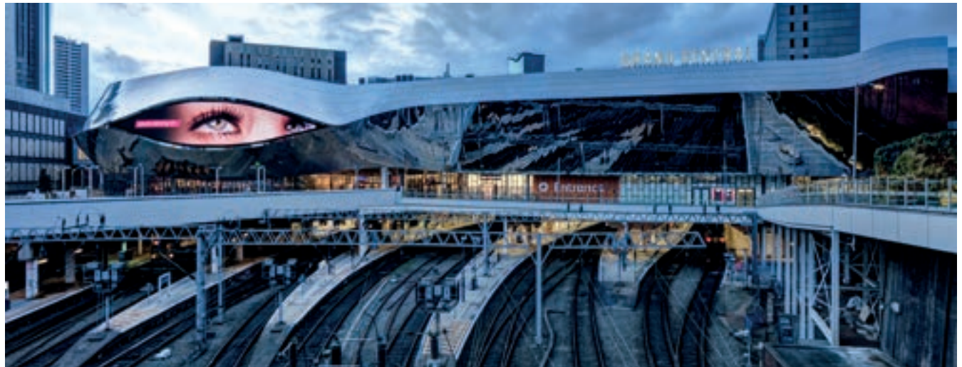
Image 6.1 Birmingham New Street facade © Network Rail
