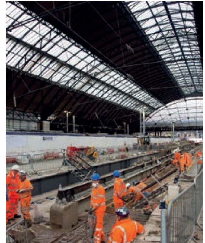
Image 9.1 Glasgow Queen Street platform extension works © Network Rail
