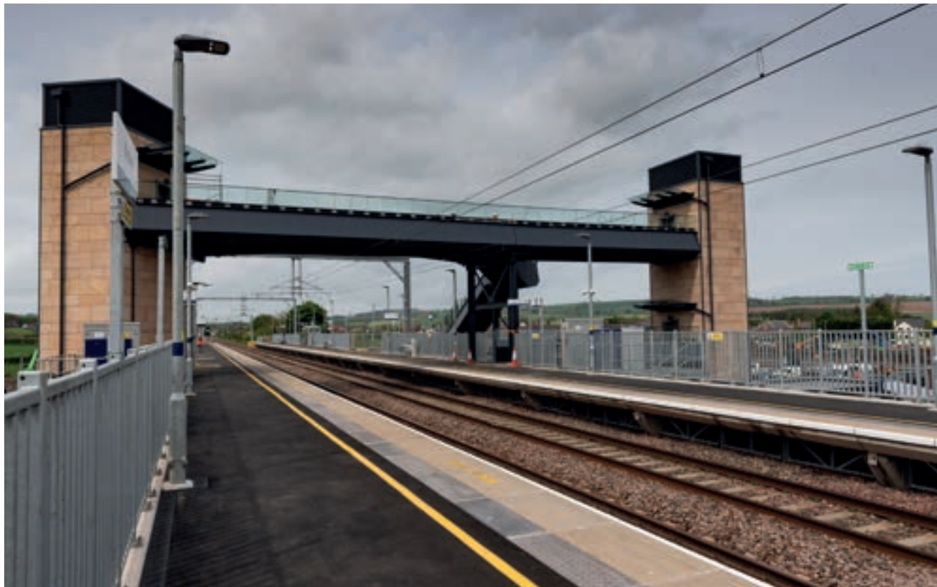
Image 4.5 Reston Station ribbon footbridge with lifts © Network Rail
