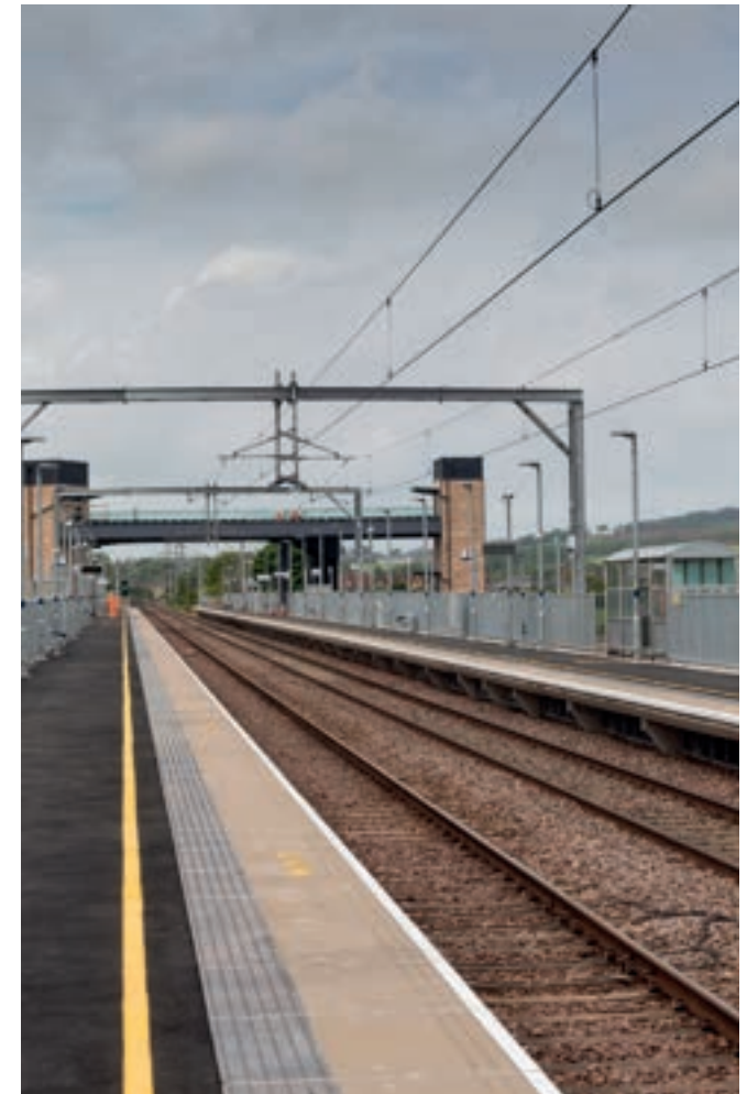
Image 10.3 Quiet platforms at Reston Station © Network Rail
