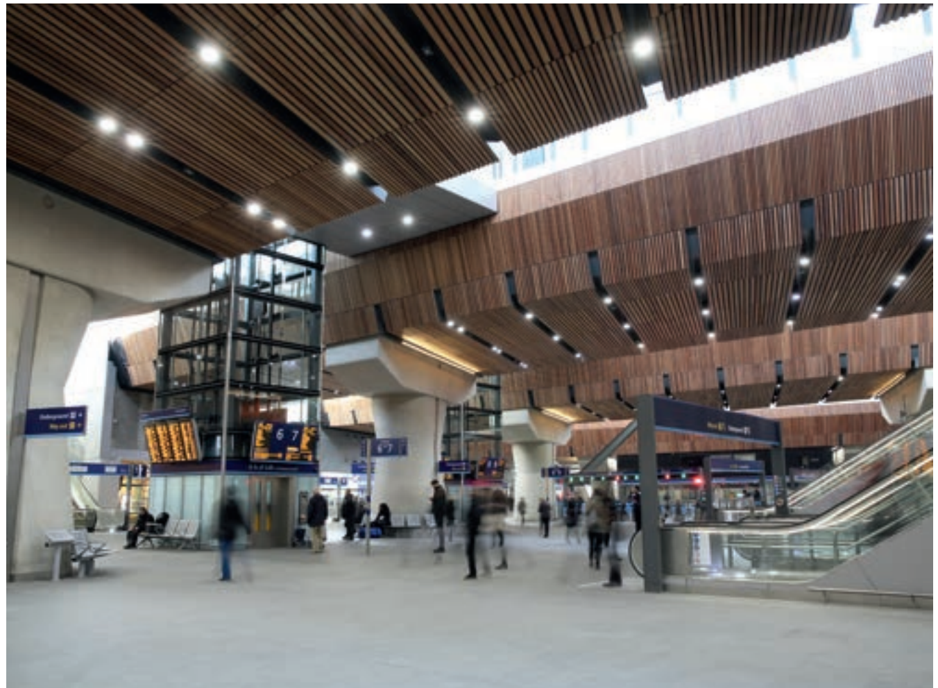
Image 5.2 London Bridge Station concourse with timber ceiling linings © Network Rail
