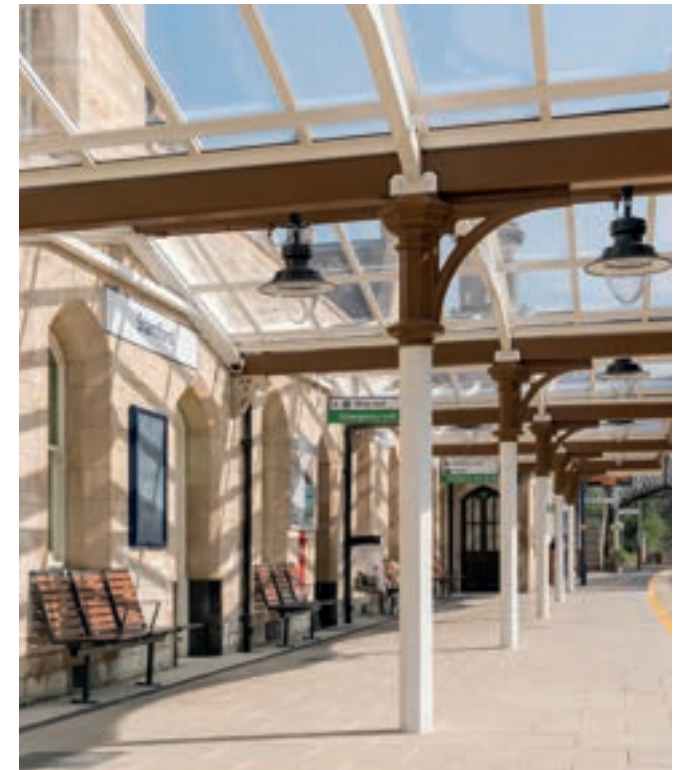
Image 5.4 Platform canopy at Stamford Station © Network Rail
