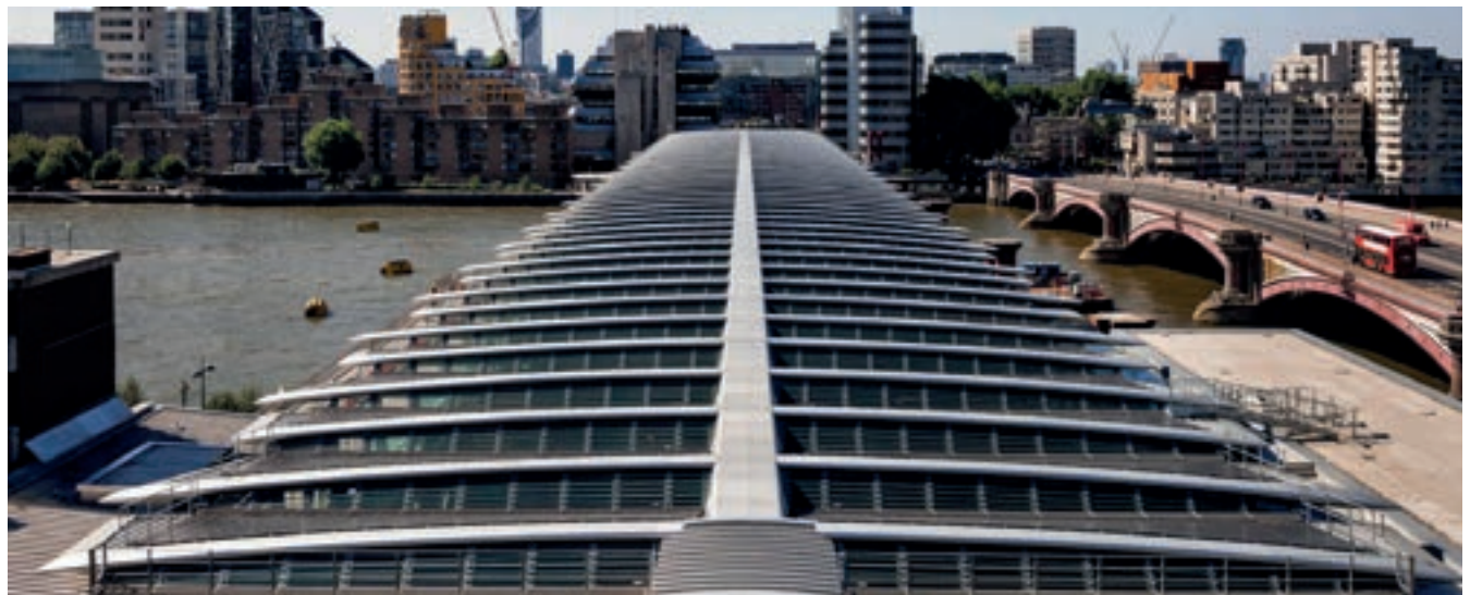
Image 6.2 PV panels on Blackfriars Station roof © Network Rail
