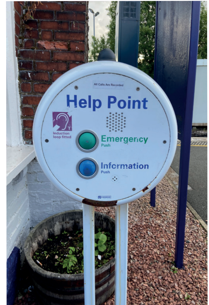
Image 8.5 Emergency Help Point © Arup
