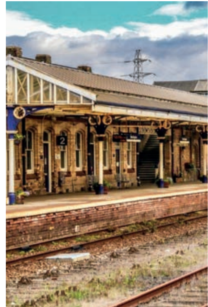
Image 1.5 Workington Station © Network Rail
