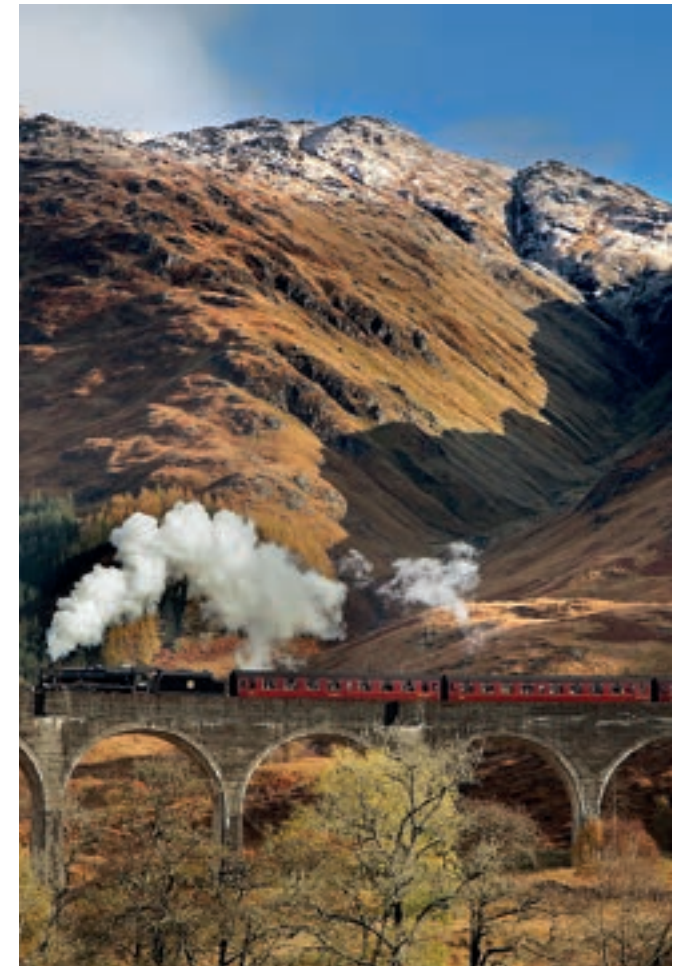
Image 1.6 Glenfinnan Viaduct, Scotland © Malcolm Blenkey. There are key differences to the statutory approval process for Scotland.
