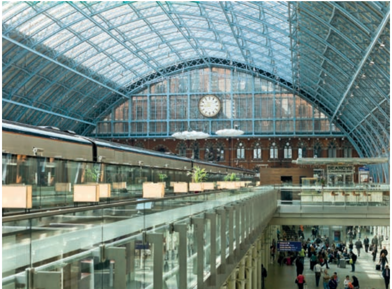
Image 3.1 St Pancras Station © Arup
