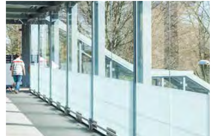
Image 3.9 Transparent glass with lower section obscured.
