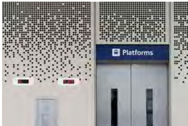
Image 3.6 Metal Cladding panels in Paddington Station
