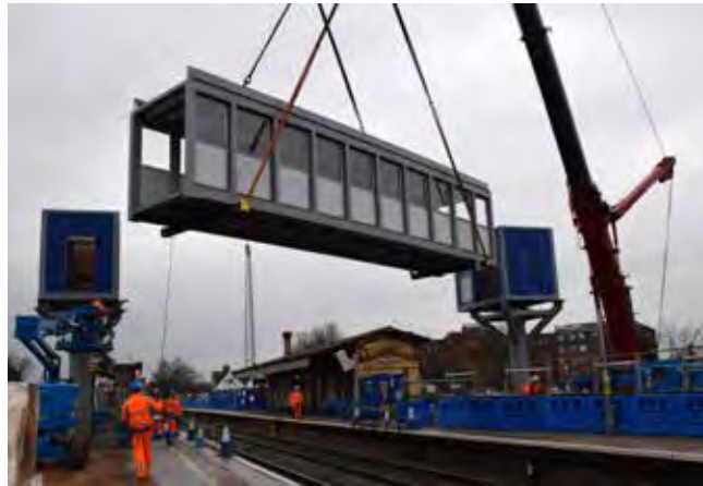
Image 2.23 Footbridge element being connected to pre-installed base elements at West Drayton station
