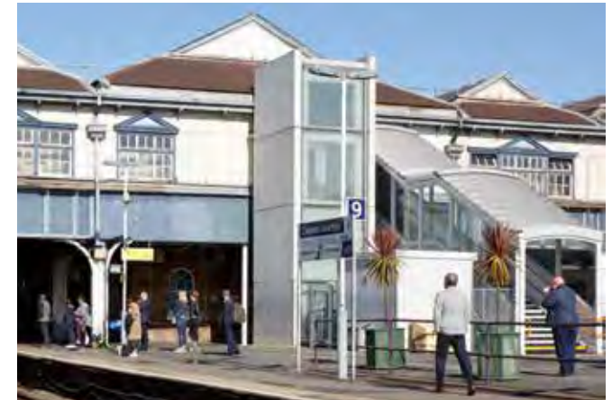
Image 2.7 Modern materials and detailing At Clapham Junction station lift shafts and new staircases have been fitted to the existing footbridge.
