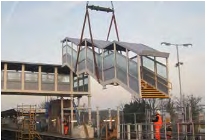
Image 2.22 Staircase being craned into place at Sittingbourne station
