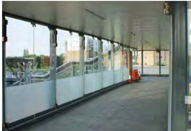
Image 2.15 Cambridge station — inwardly openable glass panels
