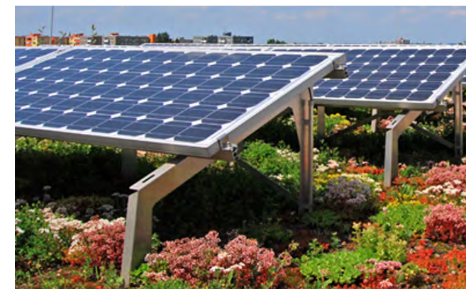
Figure 26. Building integrated solar PV installation above a green roof. Source: ZinCo Green Roof
