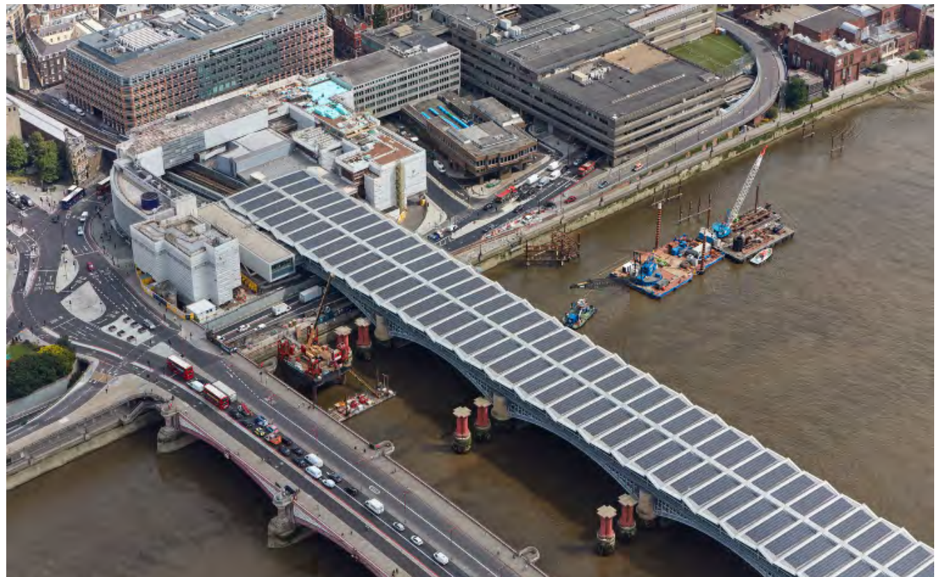
Figure 27. Solar panels on Blackfriars Station. Source: Volker Steven
