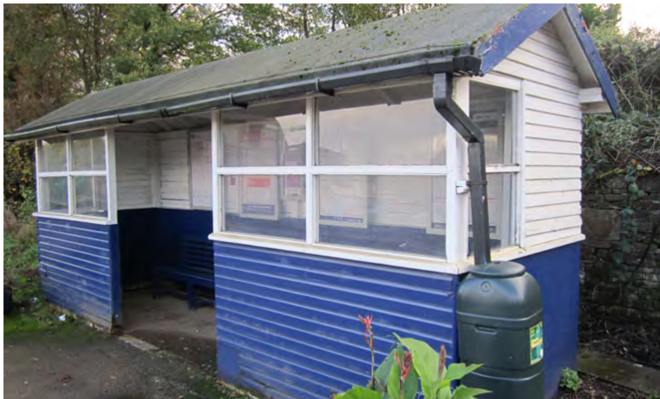
Figure 25. Gathurst station showing water butt connected to downpipe from platform shelter.
