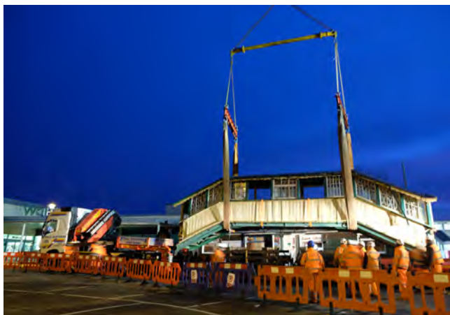
Figure 43. Alton station footbridge was deconstructed, restored and reused. © Stephen Lewis of FAS
