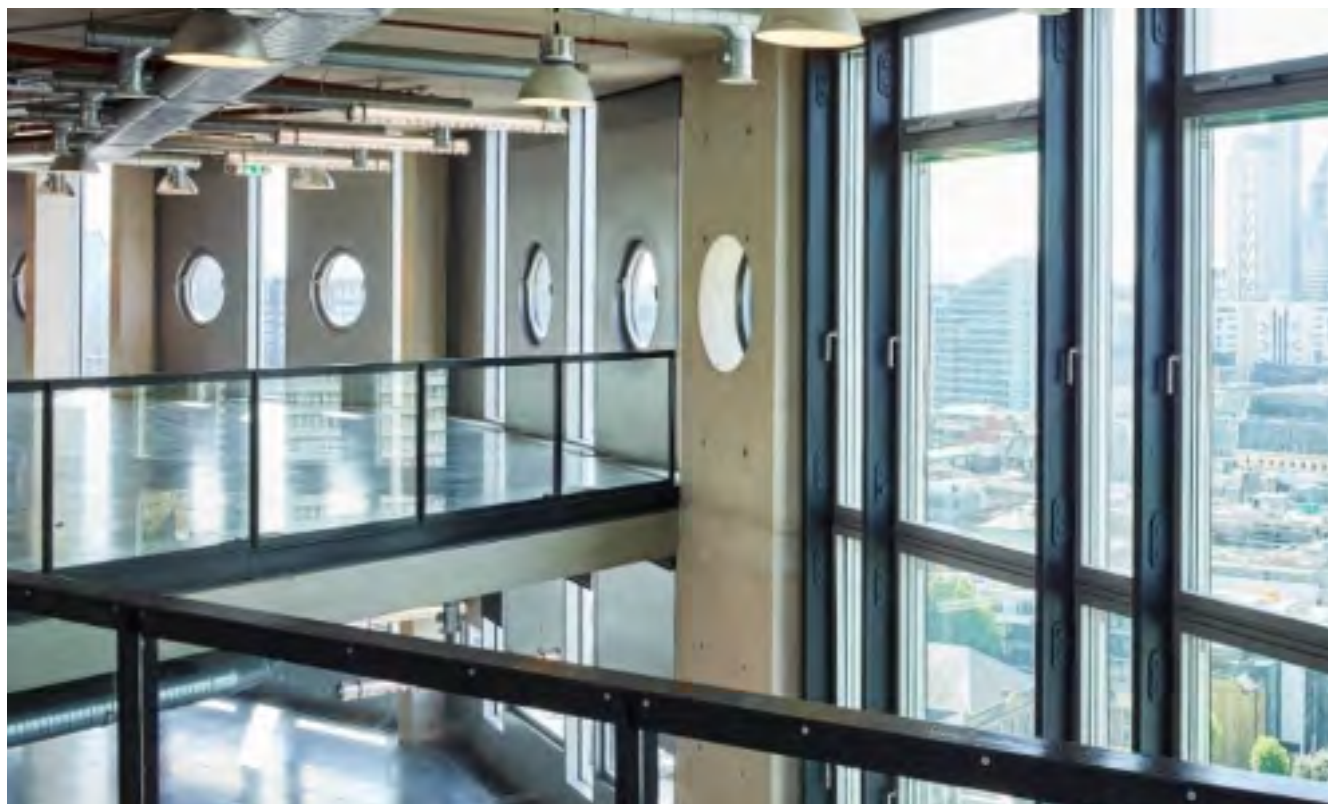
Figure 24. White Collar Factory has a mixed-mode ventilation system with user feedback as to when windows should be closed. Source: Tim Soar
