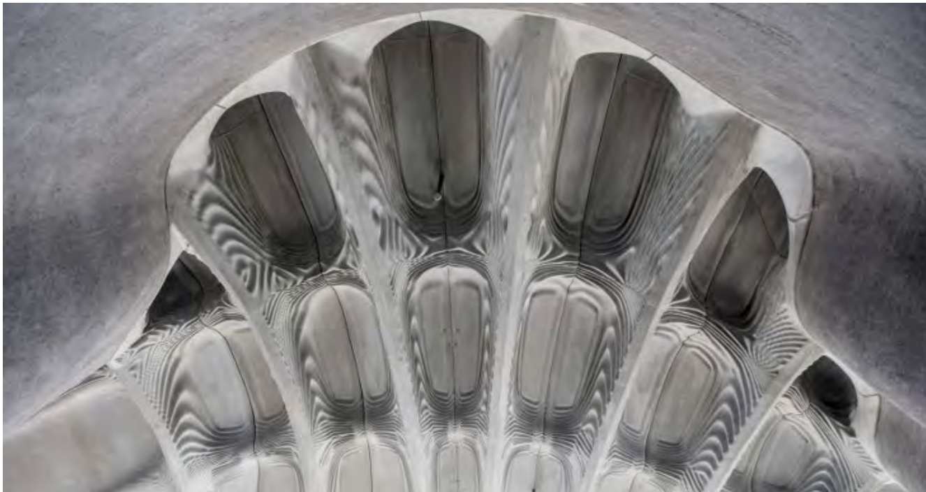
Figure 34. Digitally fabricated, precast and post-tensioned slabs allow limited depth solutions for constrained sites. The Smart Slab is a proof-of-concept requiring further development prior to widespread adoption. Source: Andrei Jipa, Digital Building Technologies, ETH Zurich
