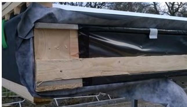
Figure 40. Timber cassettes can be delivered to site in large sizes with insulation, internal and external finishes already fixed, accelerating construction programmes. Source: Arup
