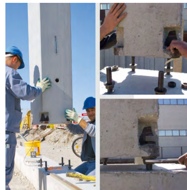
Figure 33: Precast concrete structures should be used only where other materials have been ruled out. Reversible mechanical connections should be used and high strength grouted stitches should be avoided 37 . Source: Peikko
