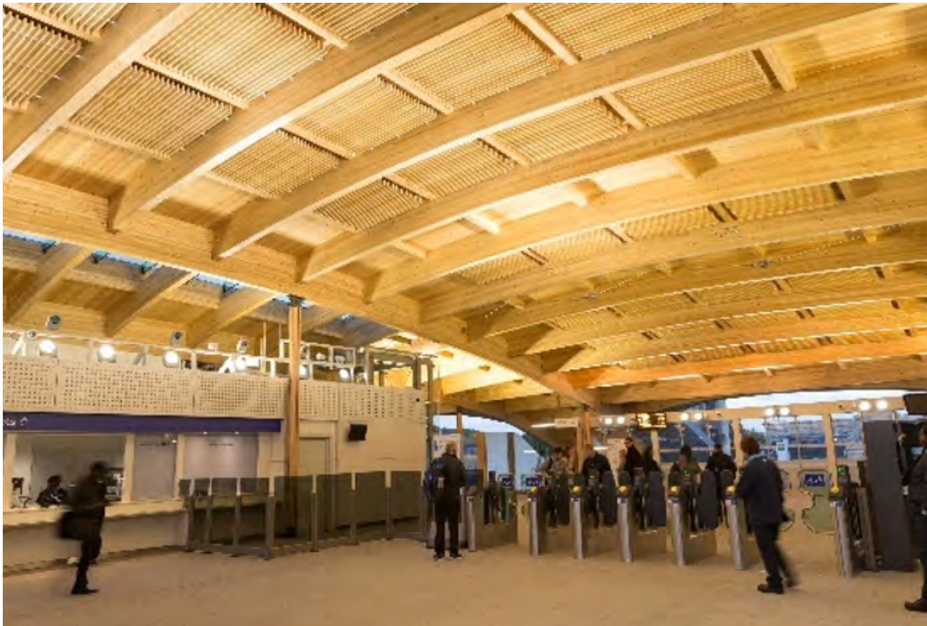
Figure 39. Abbey Wood station roof, an engineered timber beam grid which requires continuous artificial lighting as natural daylighting has not been provided for. Source: Network Rail
