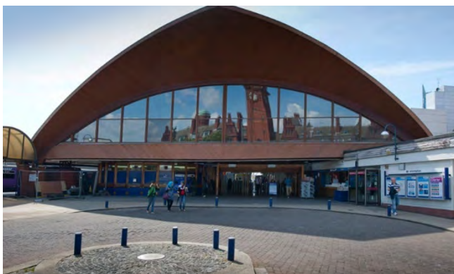
Figure 37. Manchester Oxford Road station roof, an engineered timber shell. Source: Giles Rocholl Photography
