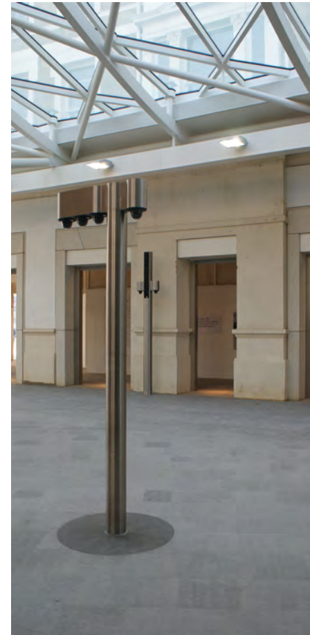
Image 6.9: Examples of elegant CCTV mounting in London's King Cross
