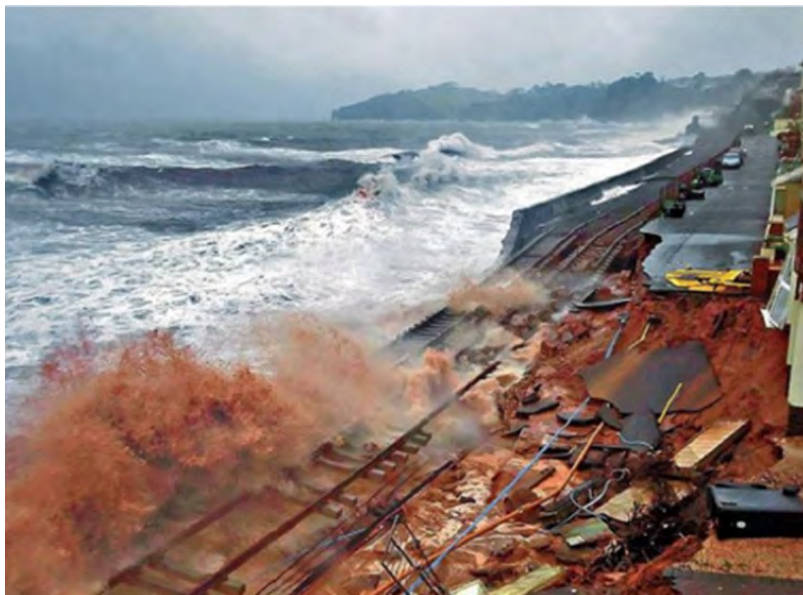
Above: The storm damage to the railway at Dawlish in 2014 and, right, just below Woodland Avenue, between Parson's Tunnel and Teignmouth
