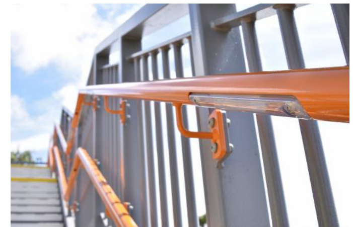
Image 3.17 Example of lighting integrated into the underside of a handrail
