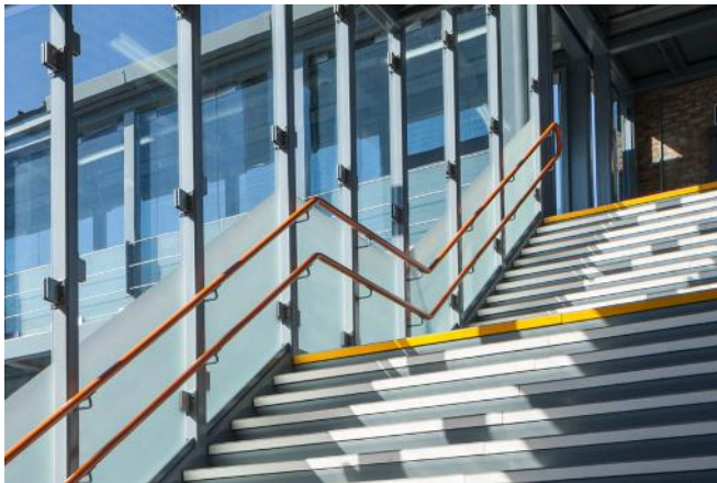
Image 4.13 Transparent glass with lower section obscured.
