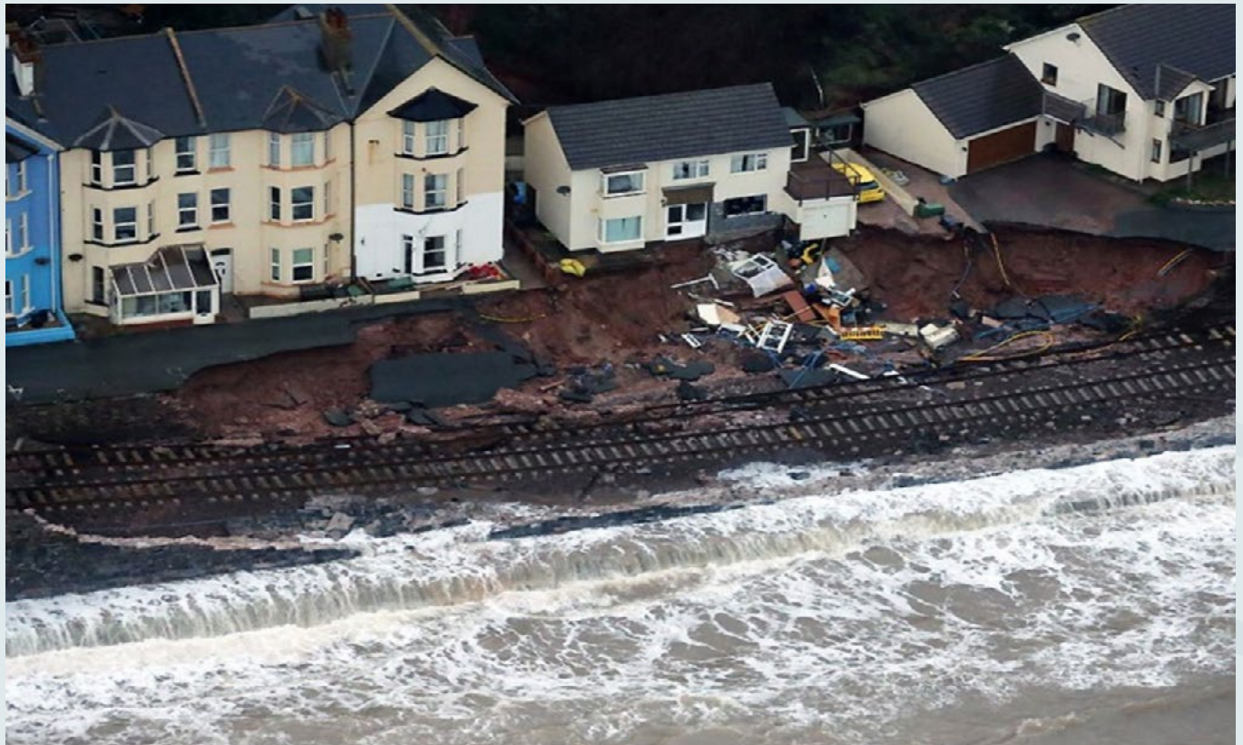
Figure 5-10 Damaged sea wall and tracks at Dawlish (2014)
