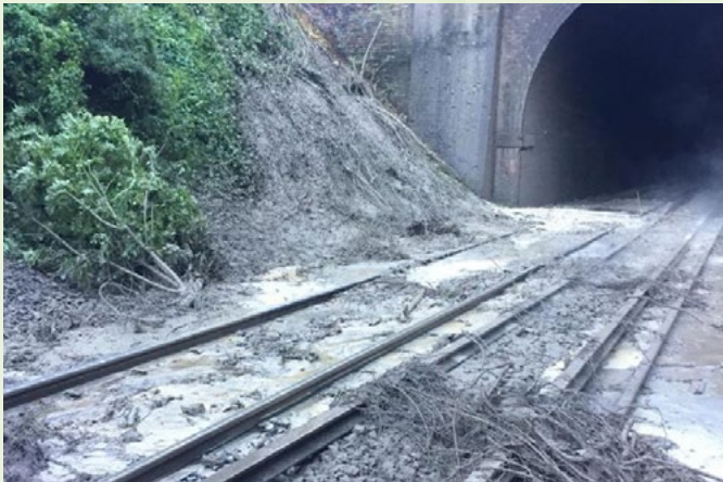
Figure 5-5 Failed Earthwork at Wallers Ash, Wessex August 2020
