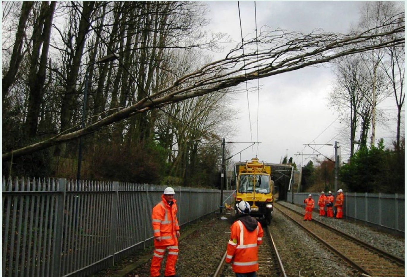
Figure 5-11 Damage to trees and OLE
