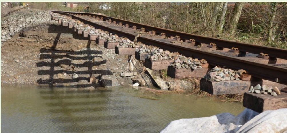
Figure 5-8 Impact of flooding from Storm Gareth (2019) on Conwy Valley line in Wales and subsequent repairs
