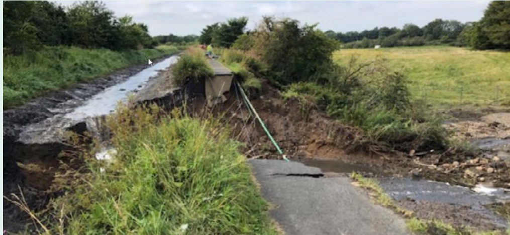
Figure 3-2 Interdependencies: the Union canal embankment collapse washed away the railway between Edinburgh and Glasgow (12 August 2020)
