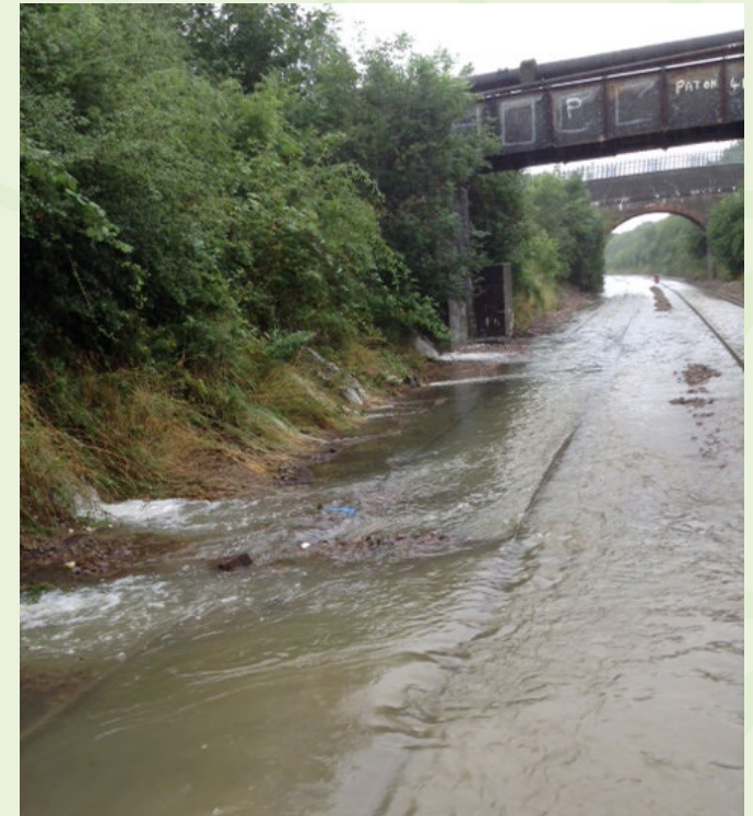
Figure 5-9 Flooded tracks at Corby in Northamptonshire, following heavy rainfall and river overflow
