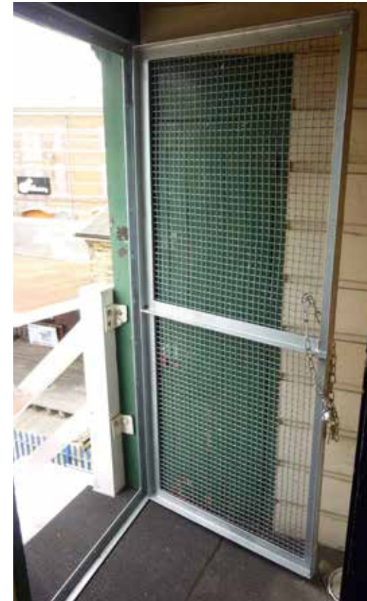
Image 4.20 Anti-vandalism measures at Canterbury East. This is a typical example of what may be considered, but a more bespoke solution may be needed at some sites. At East Holmes signal box, black grilles were required as a planning condition.
