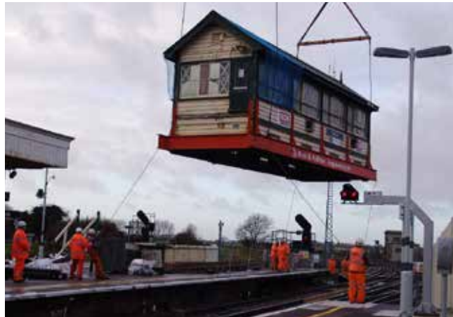
Image 4.8 Removal of Barnham signal box for relocation
