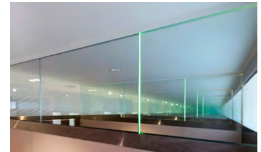
Angled panels atop cubicle walls prevents the concealment of illegal items, London Victoria WC's. Image: Peter Langdown
