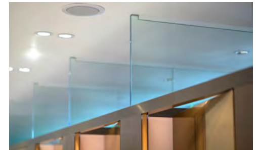
Glass dividers between cubicles, London Victoria Station. Image: Peter Langdown
