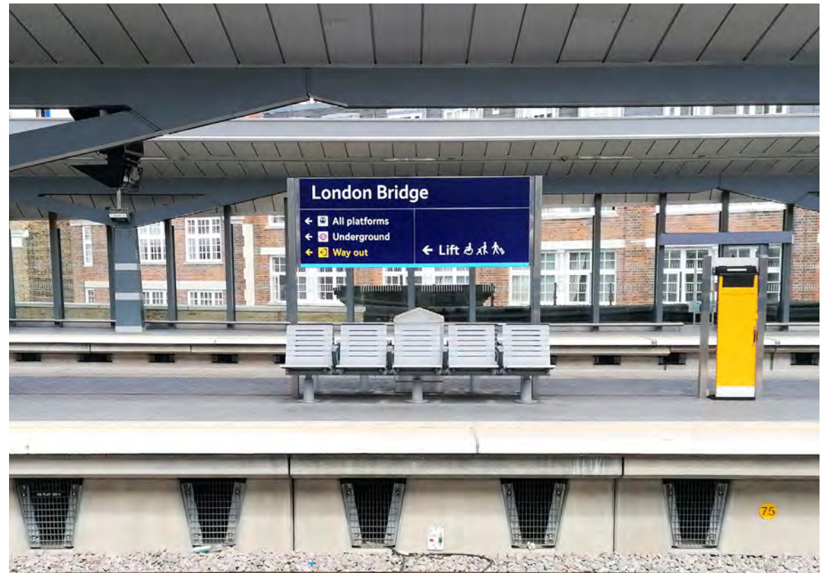
Directional platform signage, London Bridge Station. Image: Oliver Ansell
