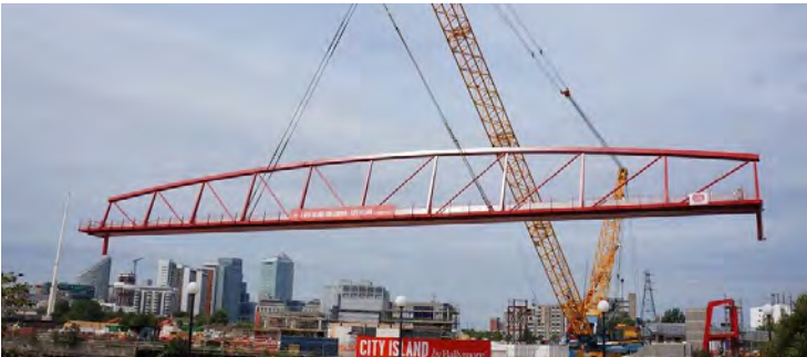
Example showing bridge lifted in to place with crane
