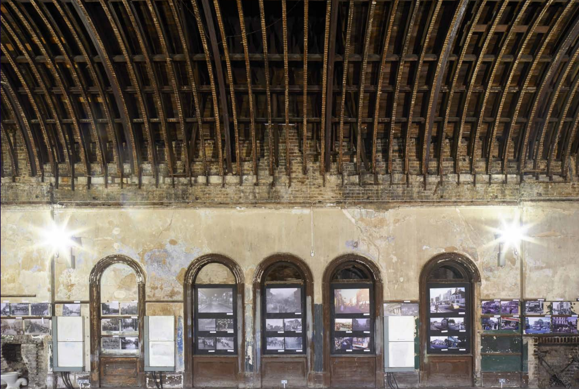
Peckham Rye Station reordering in 1935 – note how the west facing windows to the Old Waiting Room were closed, bricked up when the rear of the 'H' shaped plan was filled in with a new station platform access stair. These windows, facing Denmark Hill could be restored.
