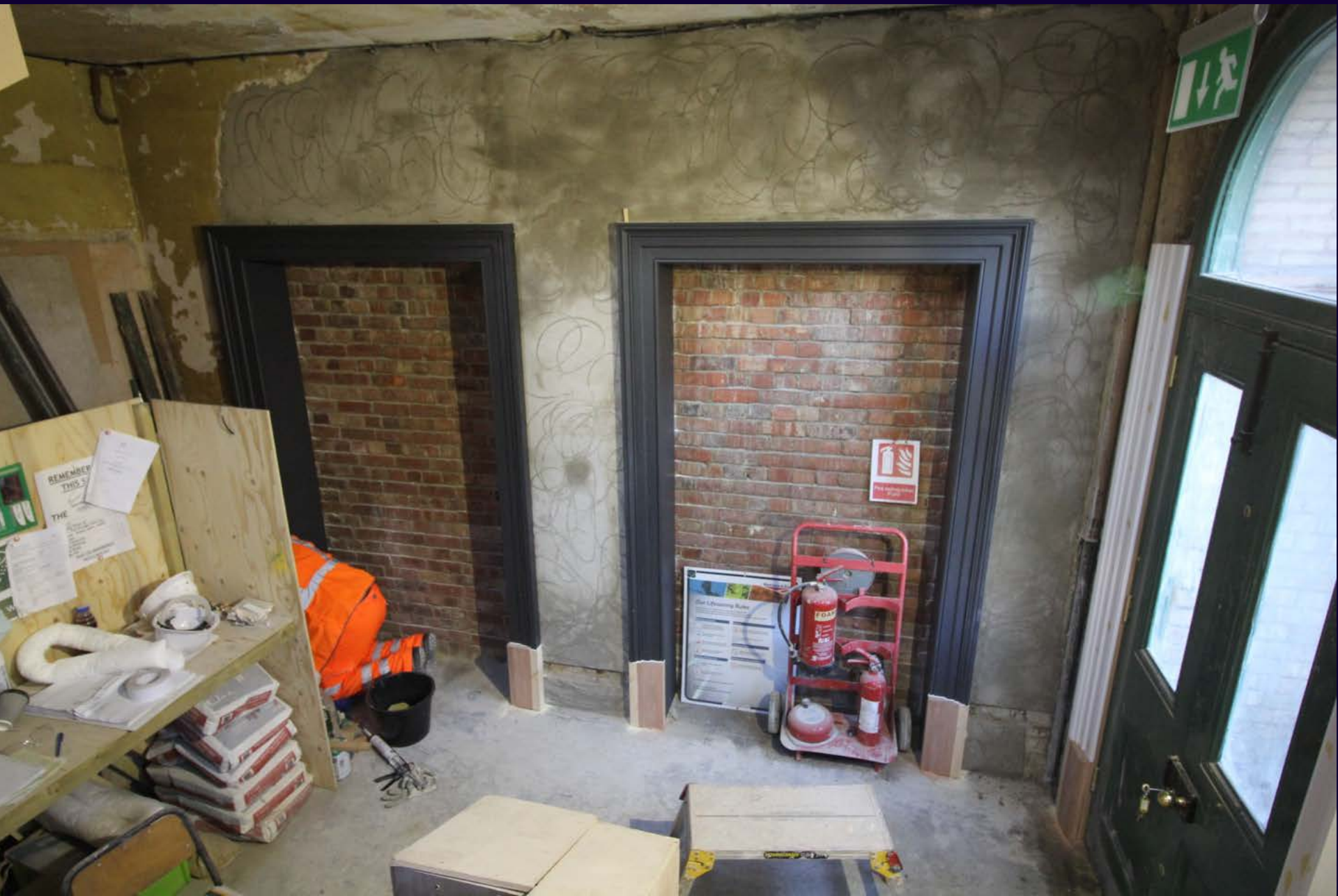
Peckham Rye Station, the South Wing & Stair restoration project, 2017. Note the bricked up doors into the Booking Hall on the ground level. The south wing stair was one of the original routes up to the platforms closed off in the 1930s when the present booking hall stair was constructed.
