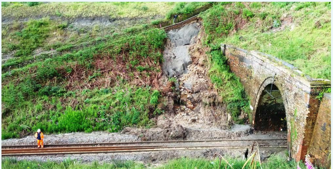
Figure 12 Honiton tunnel earthwork failure – February 2012
