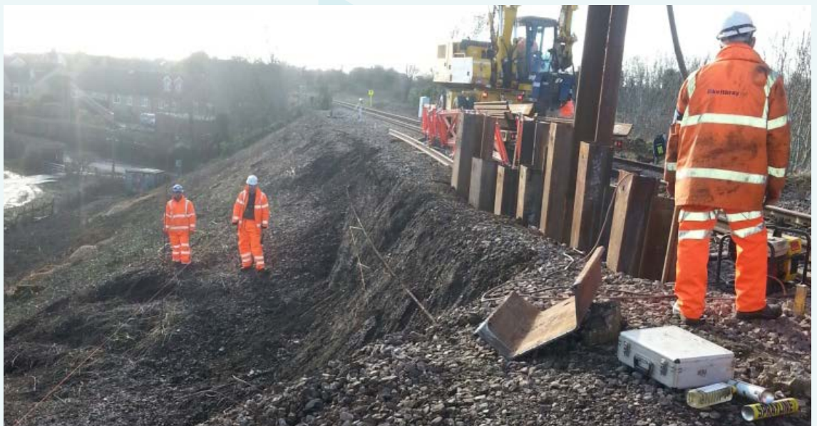
Figure 10 Undertaking temporary repairs to a storm damaged embankment at Yeovil Somerset – February 2014
