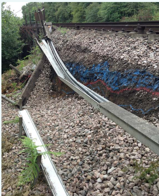
Figure 17 Pinks Hill embankment failure – July 2014
