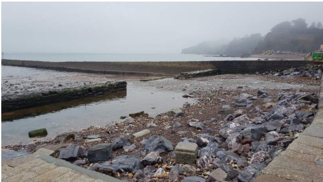
Figure 2 - Dawlish Water basin interior
