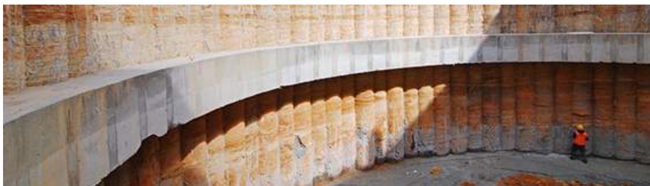
Figure 21 - Secant piled wall
