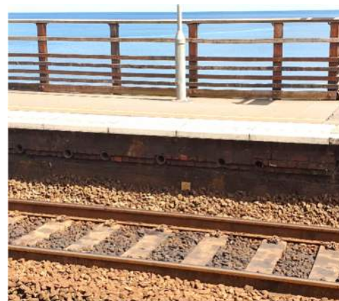
Figure 16 - High level track drainage
