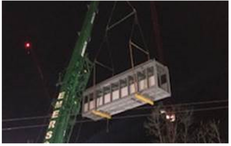
West Drayton— lifting the new footbridge into place
