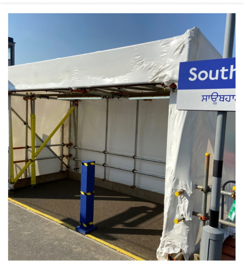
Southall - temporary rain shelter
