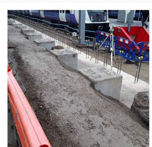
Hayes & Harlington - construction of new feature wall
