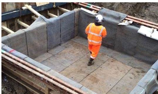
West Drayton— weatherproofing the lift shaft pits
