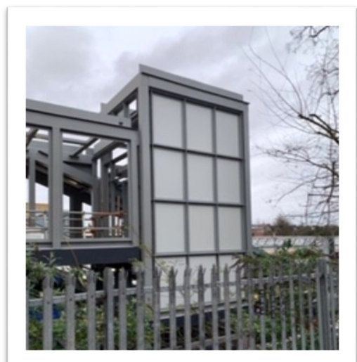
Ealing Broadway - cladding to the lift on platform 1
