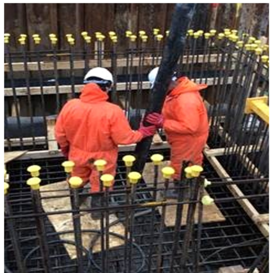
West Drayton - installing the north lift pit
