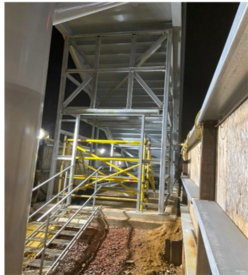
Southall - lift motor room steelwork
