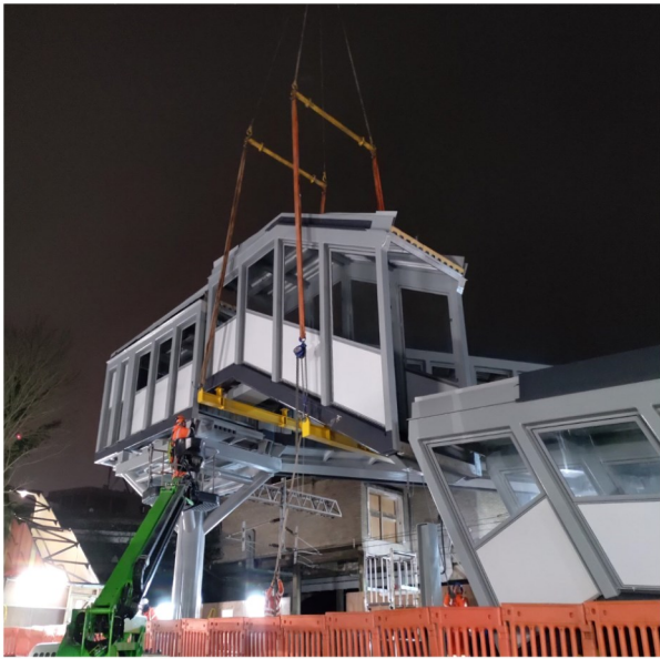
Hayes & Harlington - installing platform 1 stairs
