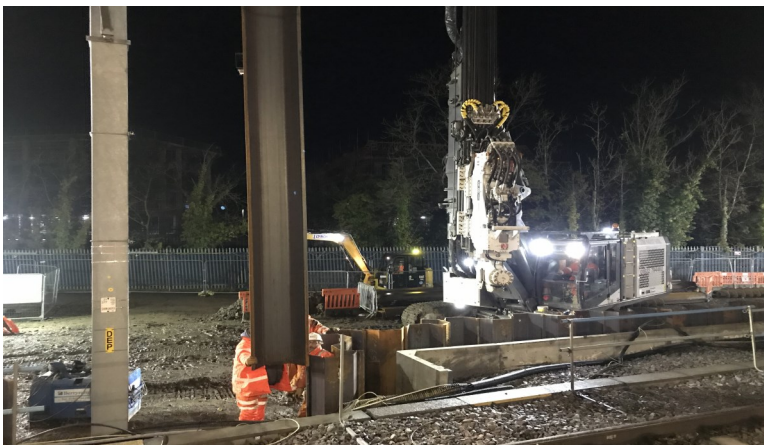
West Drayton sheet piling
