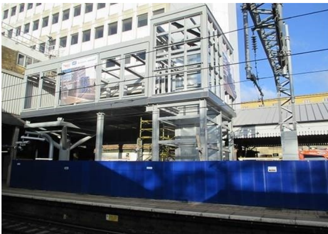
Ealing Broadway lift shafts and link lobbies
