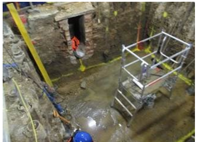
Ealing Broadway excavation of the lift pit on platform 2/3
