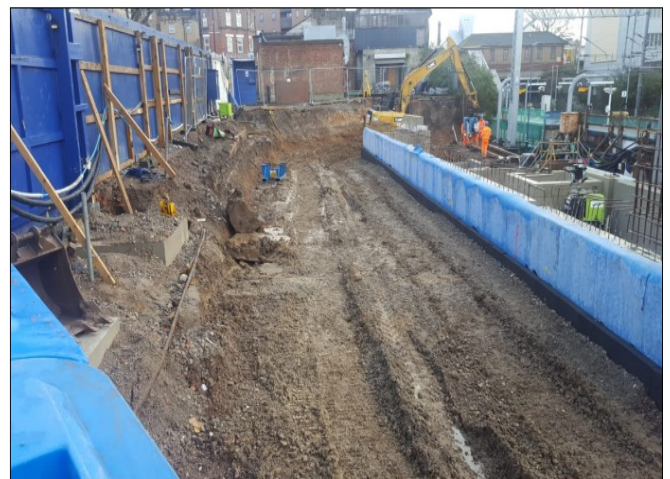
Weatherproofing the basement walls at West Ealing
