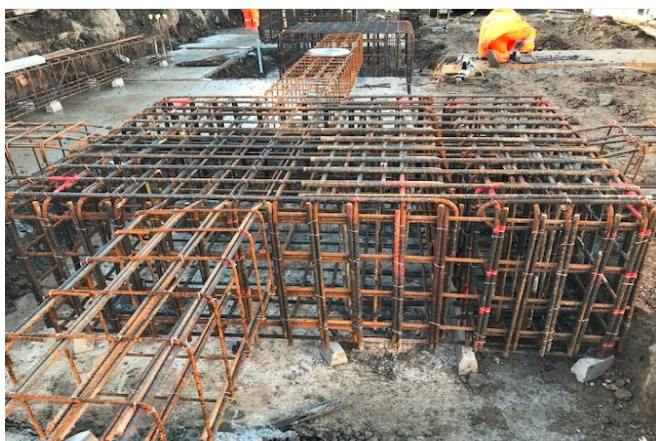
Acton Main Line preparation for ground beams
