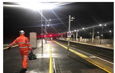
West Drayton platform extensions
