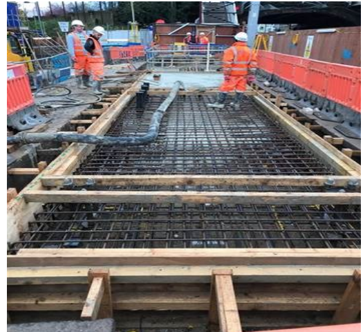
Hayes & Harlington lift foundations
