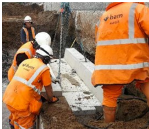
The majority of pre-cast units were installed last month
