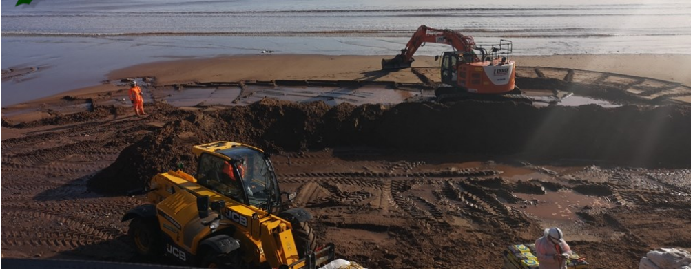
Heavy excavators are used to build sand 'bunds' to give the team extra time to carry out works
