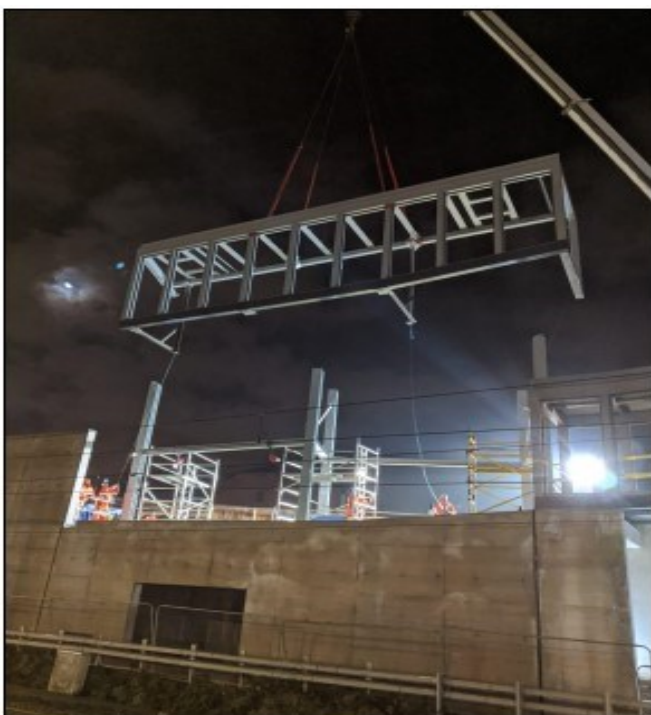
Acton Main Line—steelwork being lifted in
