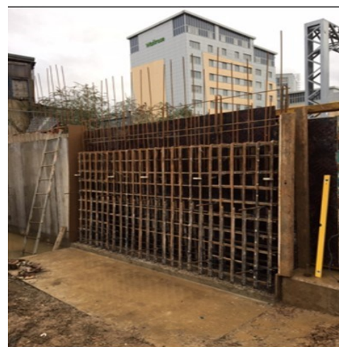
West Ealing - reinforcing steel for the East wall
