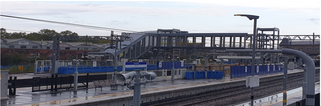
Steelwork at Southall
