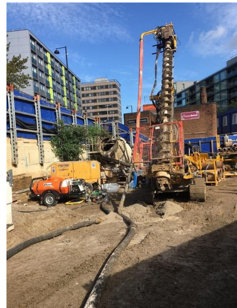
Piling works at Hayes & Harlington
