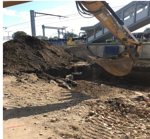
West Drayton—removing obstructions
