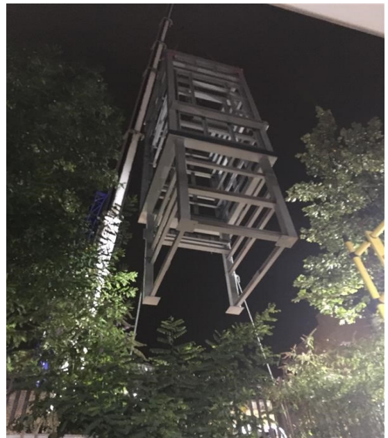
Lift shaft on platform 1 at Ealing Broadway
