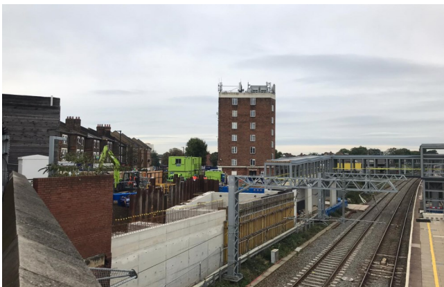
Acton basement walls
