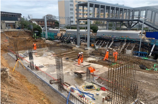
Basement foundations at West Ealing
