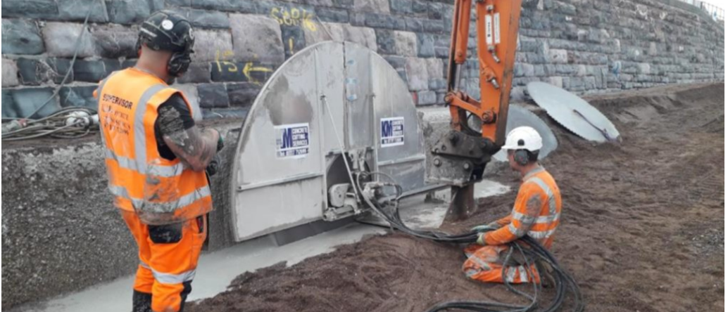
A saw cutter being used on the existing toe protection to allow us to install the foundation in front of it.
