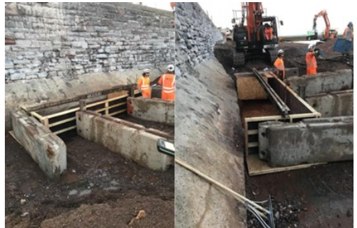
Over 60 bays are being created to form the foundation of the new wall
