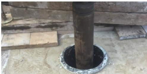
Six piezometers have been installed along the sea wall
