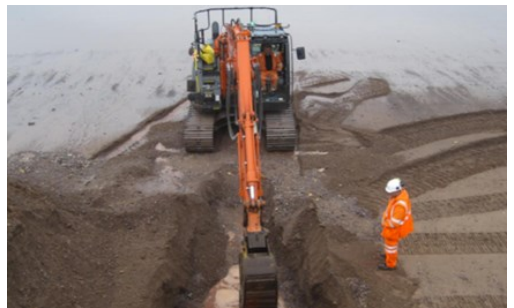
Ground investigations are being carried out
