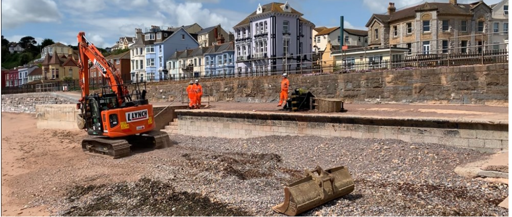
Construction on the new sea wall started on 1 June and will continue around the tides work break for the peak summer season on 14 July
