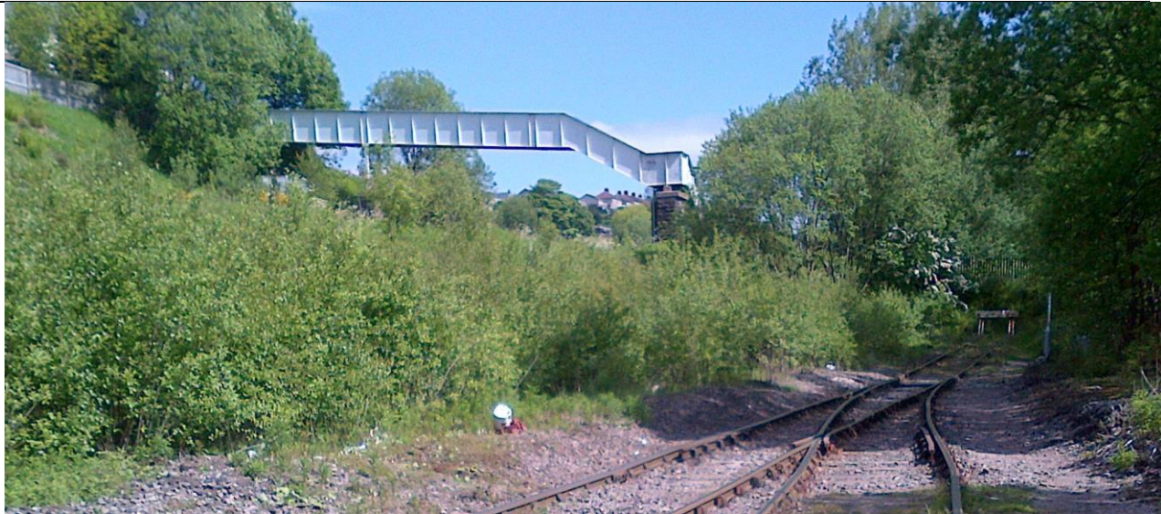
Fig.1 Existing sidings & footbridge
