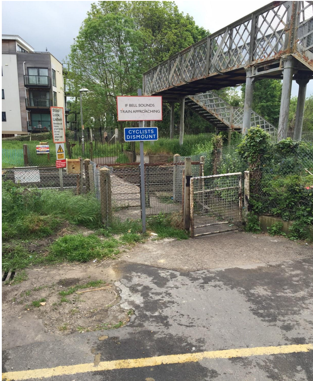
Figure 2 – Tovil footpath level crossing facing south towards Wharf Road
