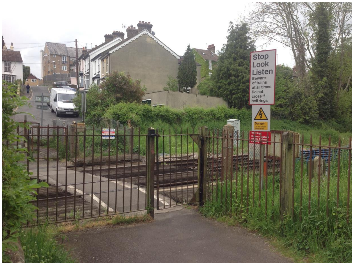
Figure 1 – Tovil footpath level crossing facing north towards Bower Lane
