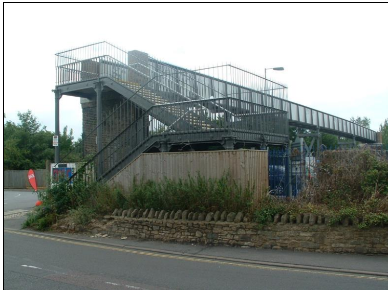
Photo 1: Eastern end of Osney Lane Footbridge at Beckett Street junction
