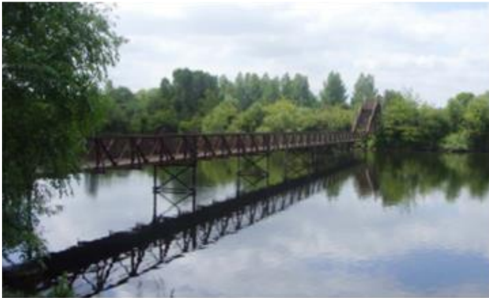
Figure 5.1.1 – Photo of Structure Crossing Hinksey Lake
