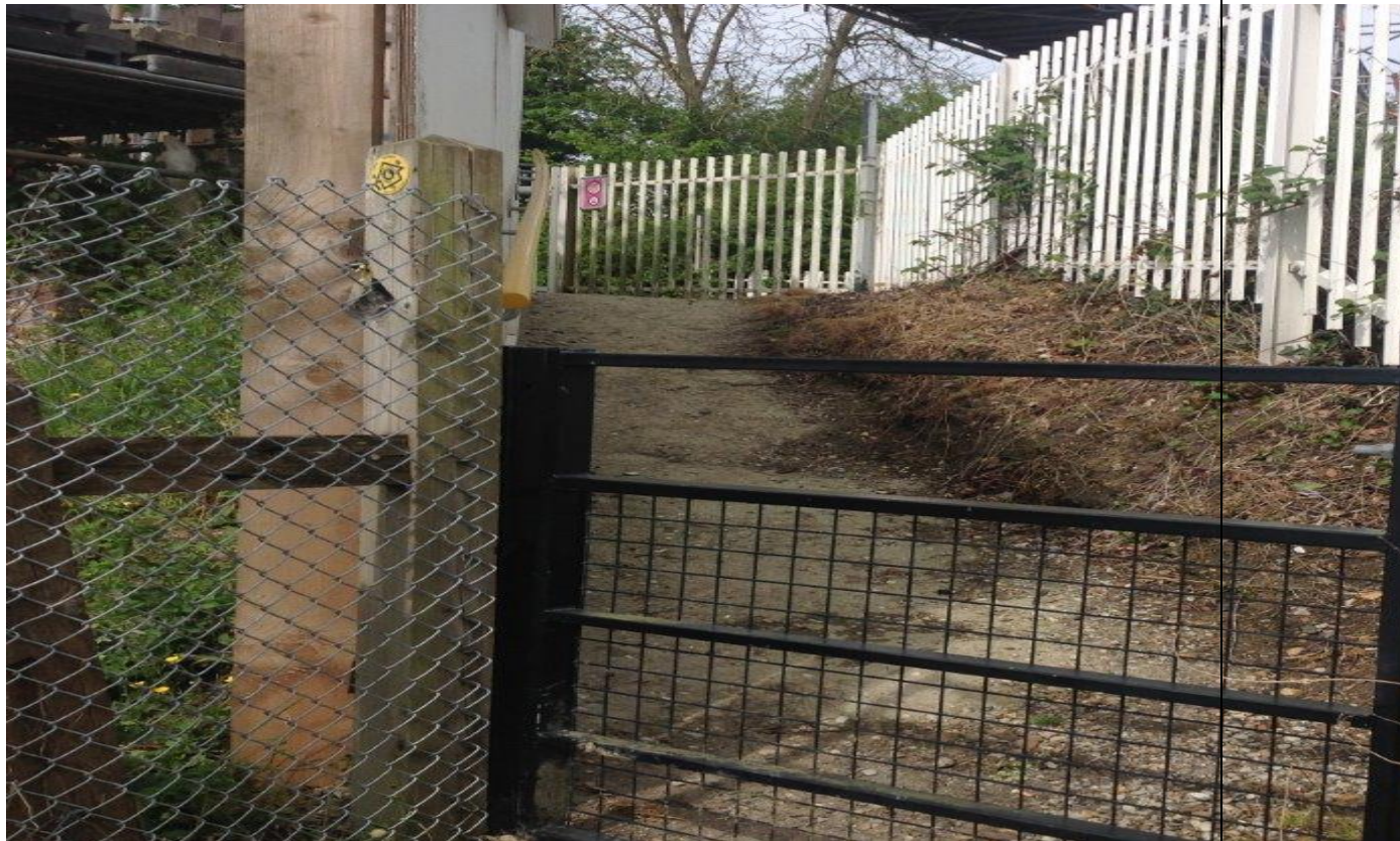
Figure 8 – PROW leading from Network Rail boundary to platform 2 (Ashford end) after the construction of temporary scaffold footbridge
