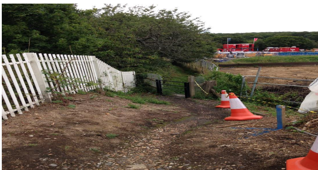
Figure 7 – PROW leading from Network Rail boundary to platform 2 (Ashford end) prior to the construction of temporary scaffold footbridge
