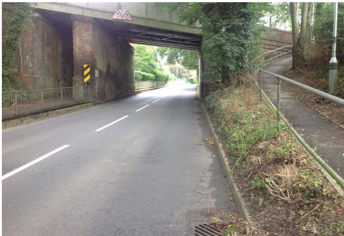
Figure 5 - Access to platform 2 (Hastings end) from Ashford Road
