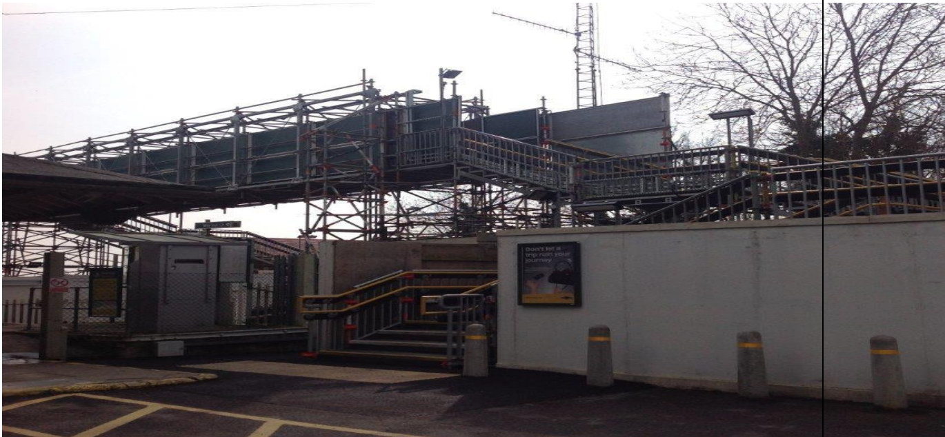
Figure 3 - Access to platform 1 (Up / Ashford International) and entrance to main station building
