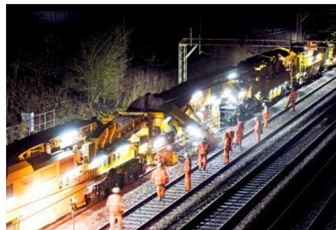
High Output ballast cleaning on the West Coast Main Line
