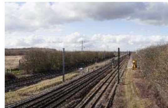
Figure 26: Grade separation works at Werrington
