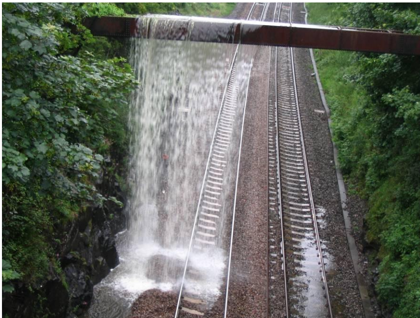
Figure 8 The overtopping of an aqueduct demonstrates the importance of understanding surrounding water systems
