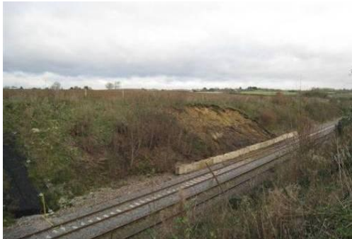
Figure 46 Landslip at Langport cutting (November 2012)
