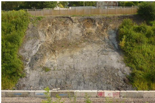
Figure 48 Slip failure at Chipping Sodbury West (2012)
