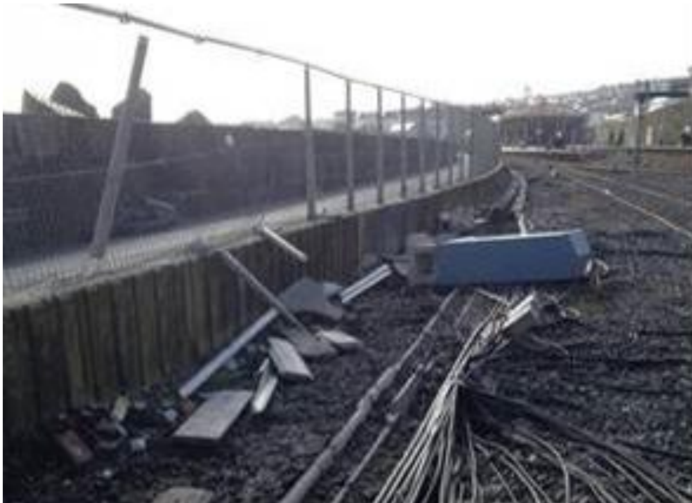
Figure 39 Signalling cables and equipment strewn across the track at Penzance after February 2014 storms
