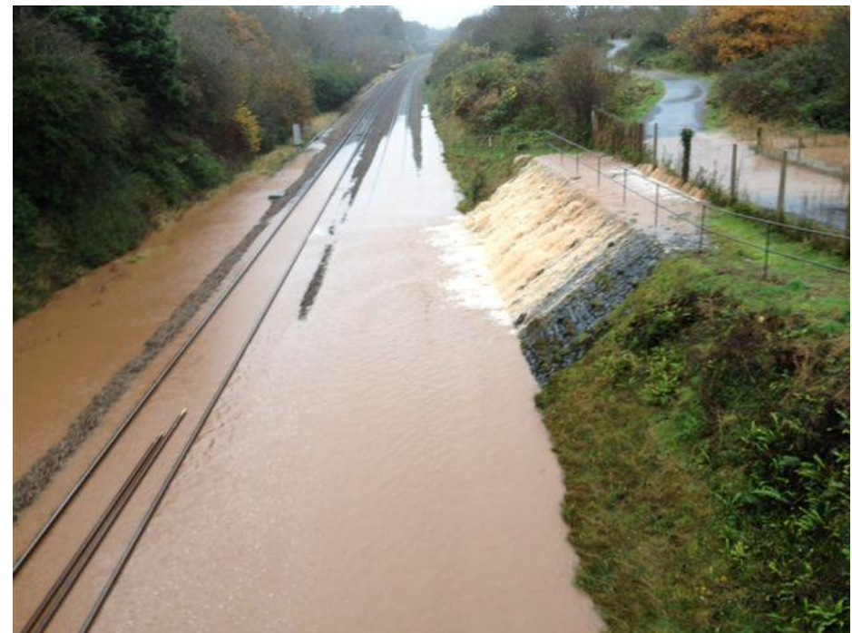
Figure 30 Surface water flooding cascades on to the track at Flax Bourton, Bristol
