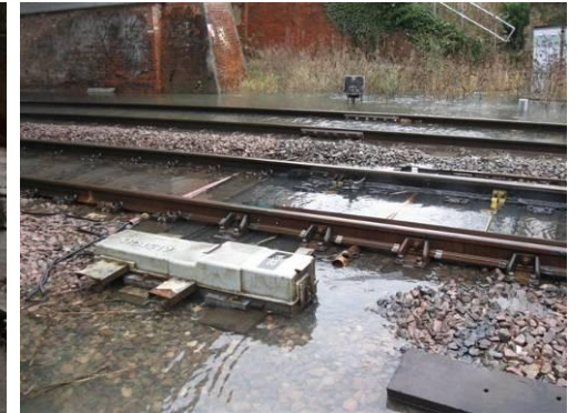
Figure 36 As well as reduced speeds, points cannot be used, reducing operational flexibility
