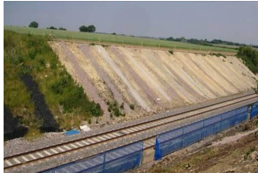
Figure 47 Remediated Langport cutting with counterfort drains (June 2013)
