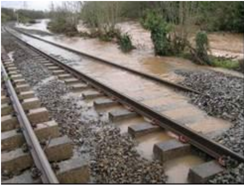
Figure 33 Water floods on to the track from the River Exe flood plain at Cowley Bridge Junction, Exeter
