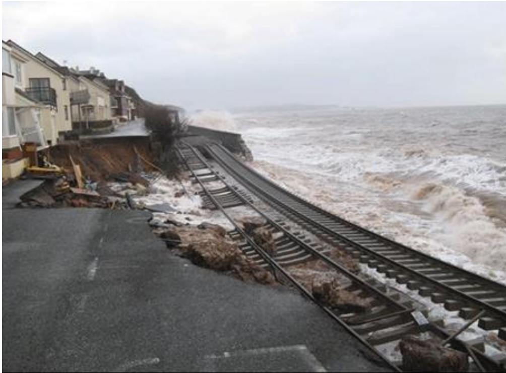
Figure 41 Suspended track and suspended train service at Dawlish following February storms
