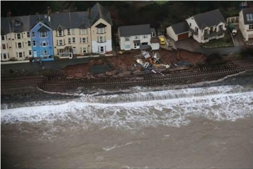
Figure 13 Dawlish sea wall breach, February 2014
