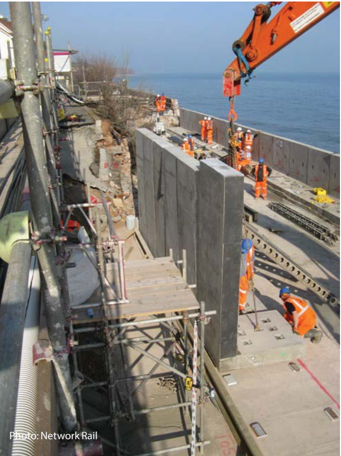
Installing concrete sections to reinforce the Dawlish seawall
