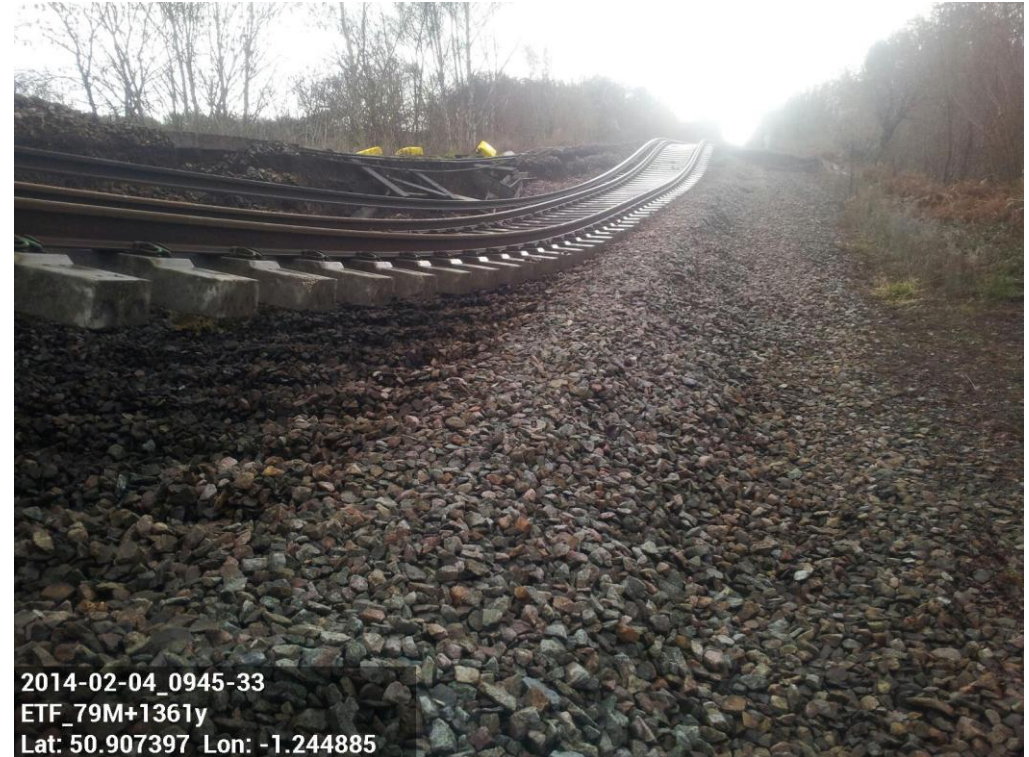
Figure 7 Earthslip at Botley following unusually wet winter of 2013/2014.
