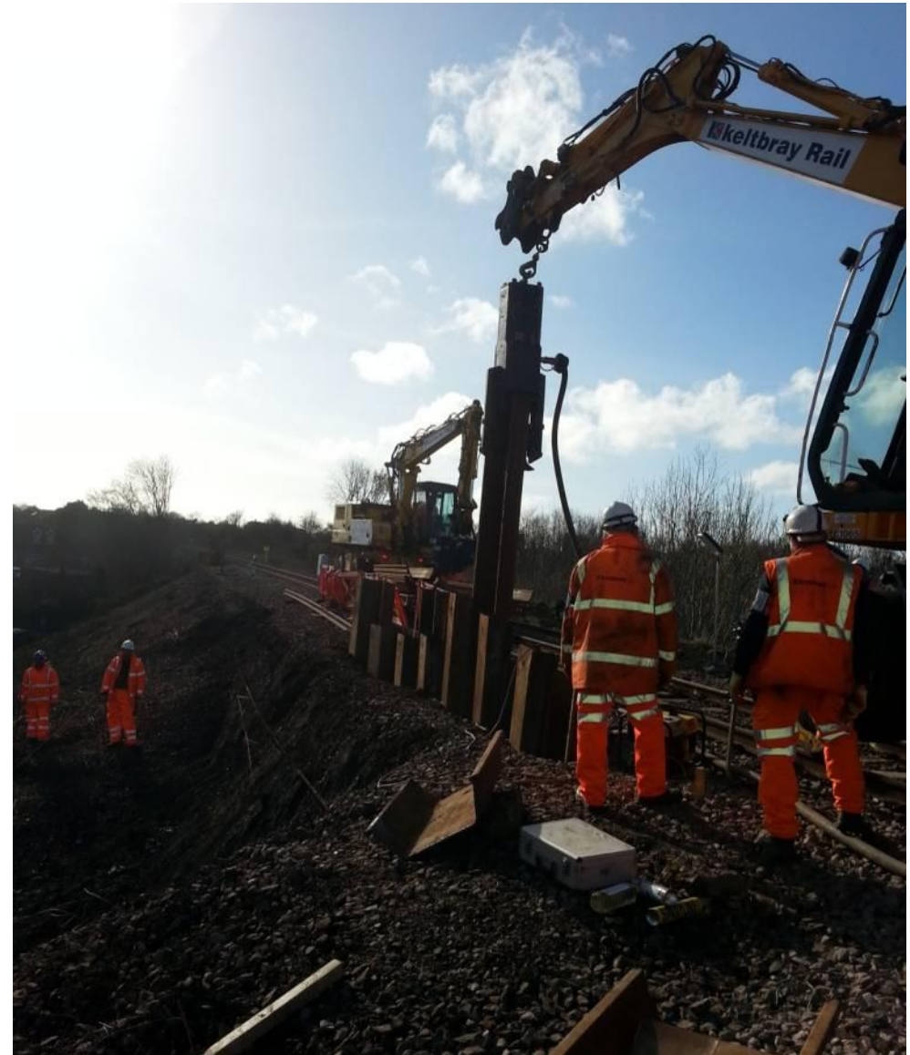
Figure 27 Undertaking temporary repairs following an embankment failure near Yeovil in the winter of 2013/2014.
