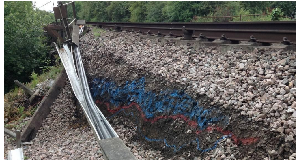
Figure 15 Pinks Hill track support failure
