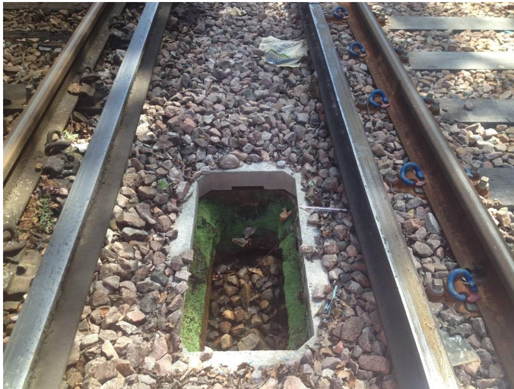
Figure 28 A typical drainage system in need of clearance and possibly replacement.
