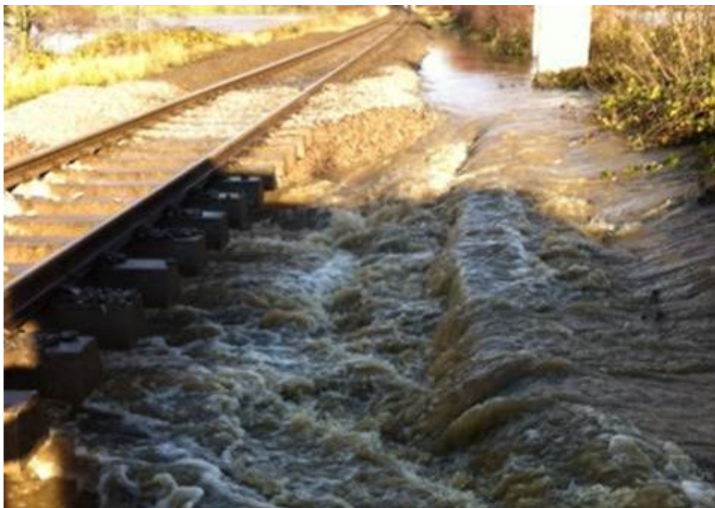
Figure 13 Track washing out at Broom near Axminster
