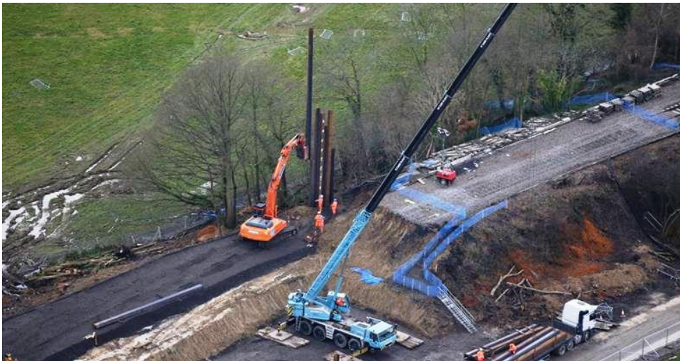
Figure 26 Undertaking repairs to the embankment at Botley following its collapse in the winter of 2013/2014.
