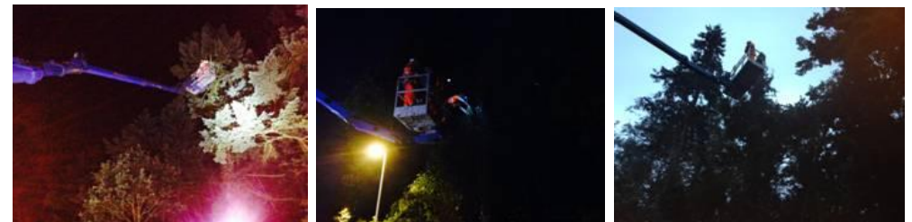
Figure 25 Staff using a Mobile Elevating Work Platform (MEWP) to reduce the height of a tree in danger of falling on to the line.
