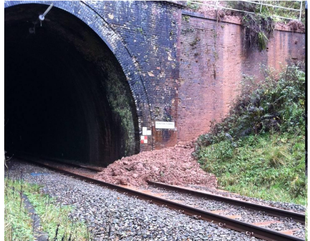
Figure 12 Honiton tunnel earthwork failure
