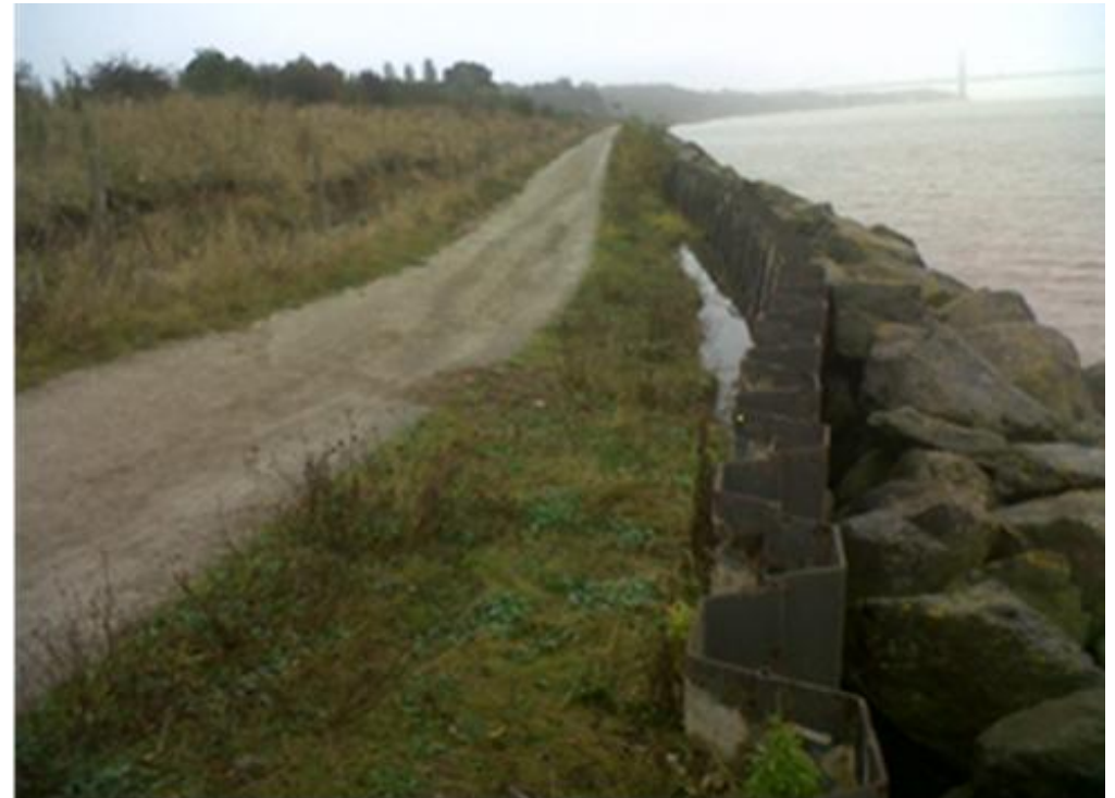
Figure 45 Hessle Foreshore sheet piled wall in October 2012
