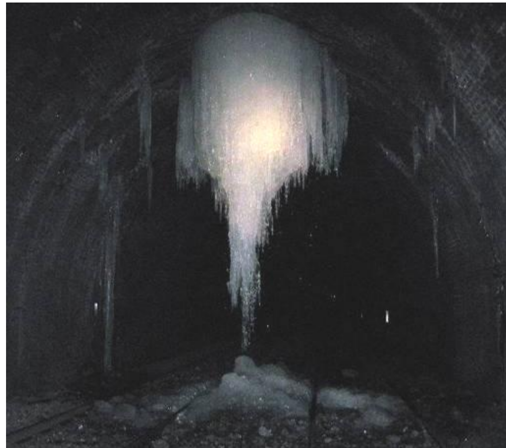
Figure 37 Tunnel shaft with frozen groundwater
