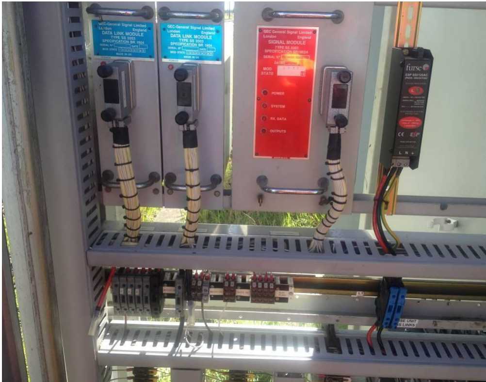
Figure 42 FURSE lightning protection installed in trackside signalling cabinet
