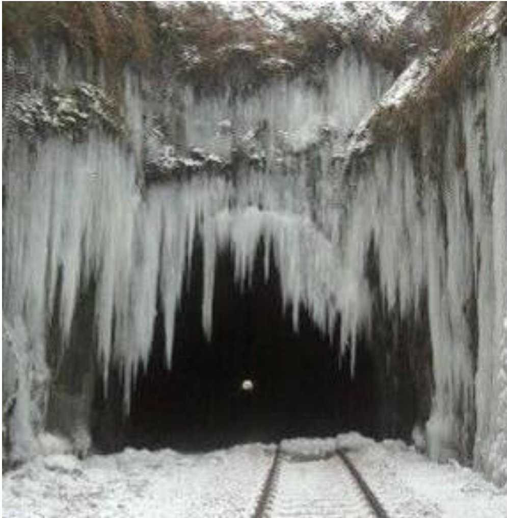
Figure 38 Tunnel portal with frozen surface water
