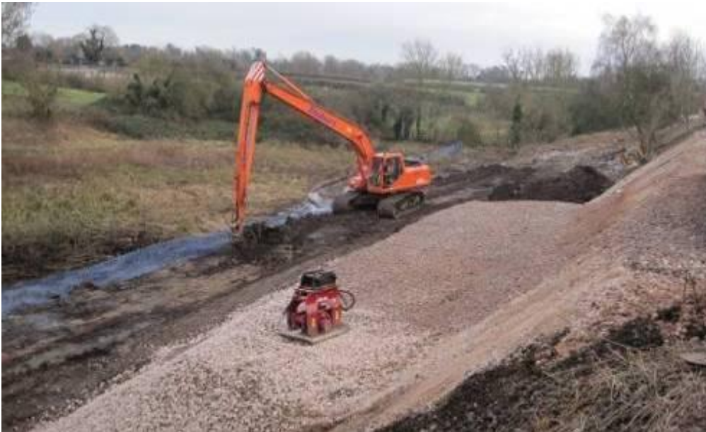
Figure 35 Barrow Upon Soar earthwork regrade
