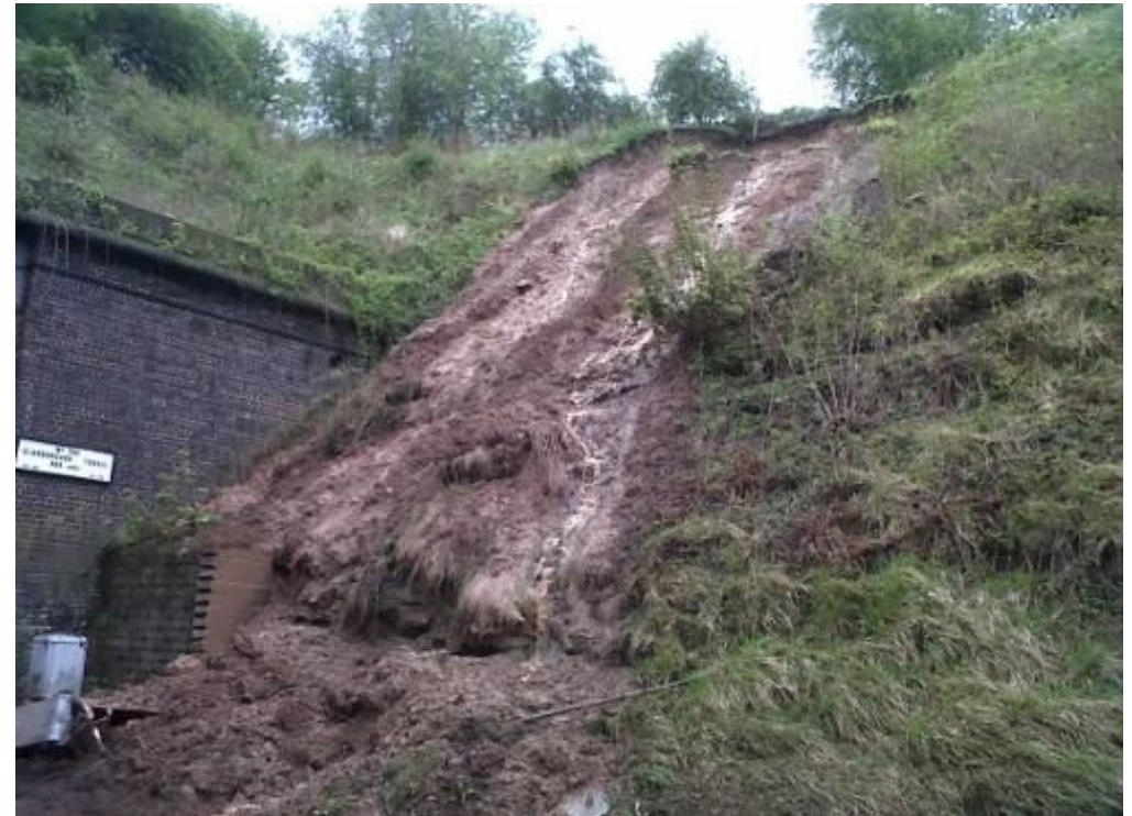
Figure 34 Clarborough tunnel failure
