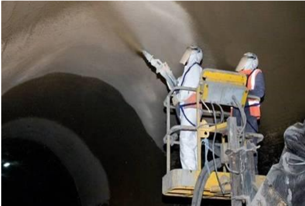
Figure 40 Spray applied structural concrete
