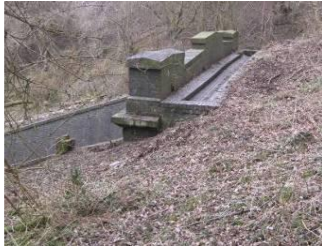
Figure 39 Tunnel portal crest drainage
