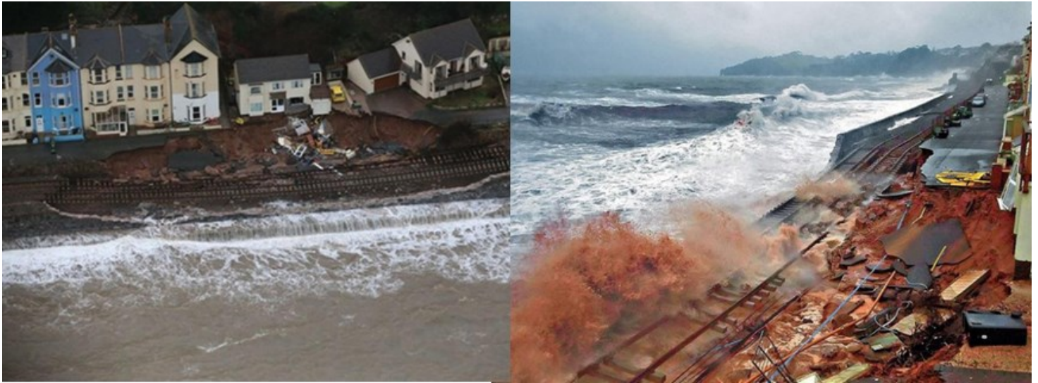
Figure 1 – Images of the breached railway at Dawlish, 4th February 2014.
