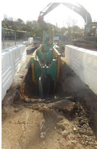
Figure 3-14: Deep cut-off trench drain under construction
