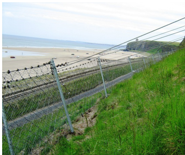
Figure 3-13: Tethered rockfall catch fence
