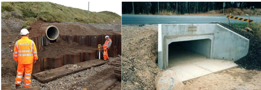
Figure 3-15: UTX drain (left) and box culvert (right)
