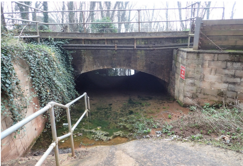
Figure 3-11: Drainage culvert beneath track at Shell Cove
