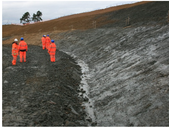
Figure 3-17: Slope regrade at Chipping Campden, 2014
