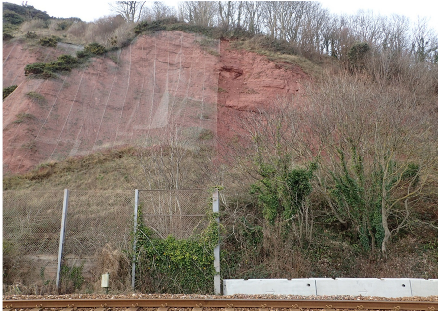
Figure 3-7: Meshing near Parson’s Tunnel
