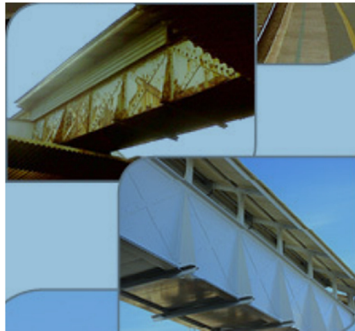
Figure 3-24: Old steel v new grp footbridge at Dawlish Station
