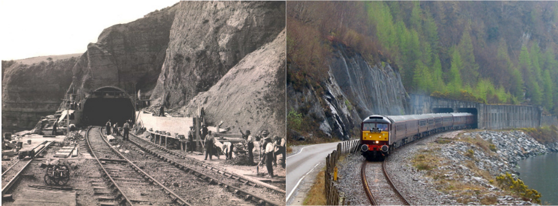
Figure 3-16: Construction of rockfall shelter at Parson’s Tunnel (1921) and near Stromeferry, Scotland
