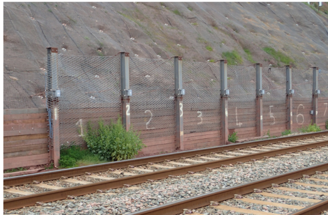
Figure 3-9: Cliff fall barrier at Woodlands (CBU10)
