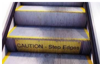
Figure 6 safety signage on escalator step
