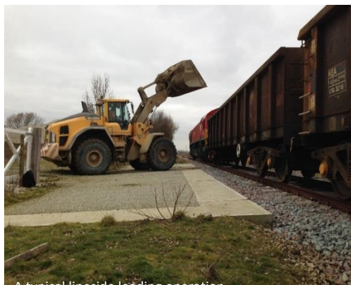
A typical lineside loading operation
