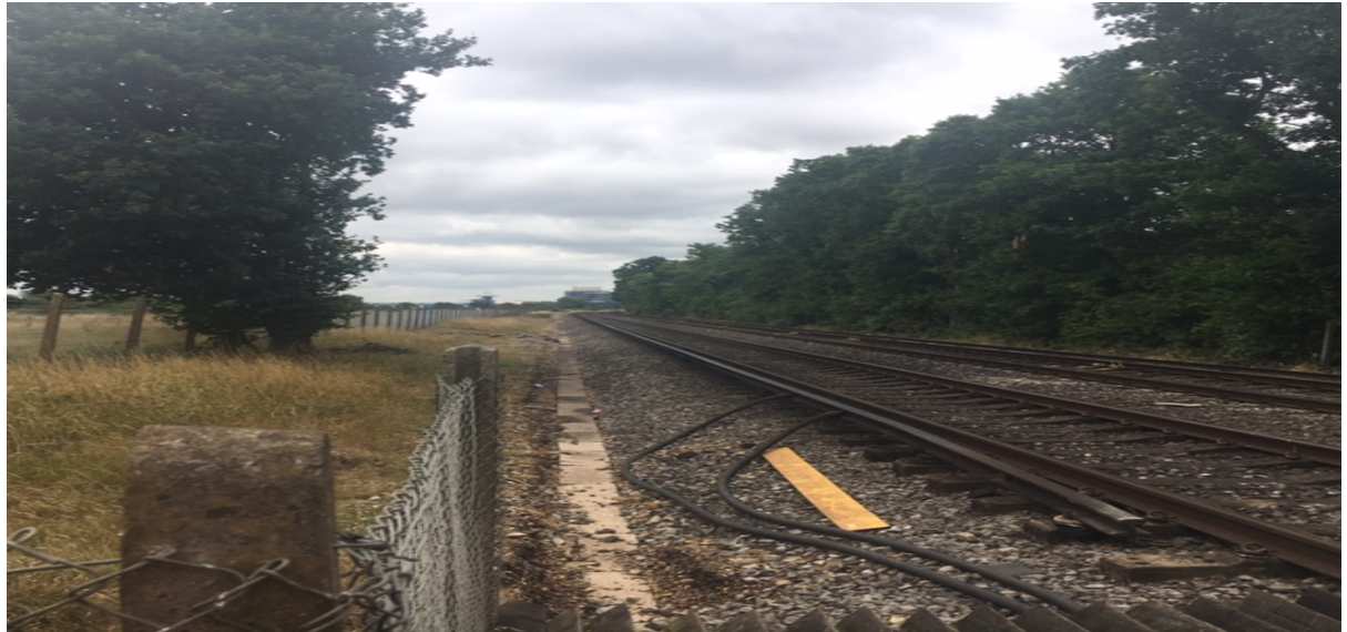
East side looking North (Down side down train approach)
