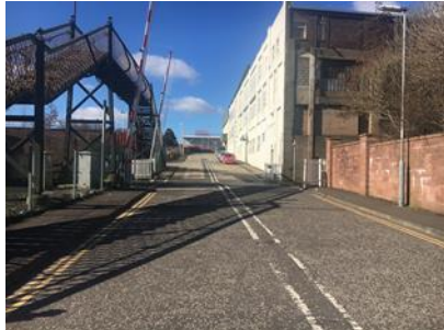
Up side crossing approach
